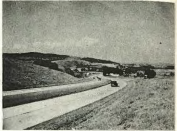
2.- RURAL NATIONAL INTERSTATE HIGHWAY
