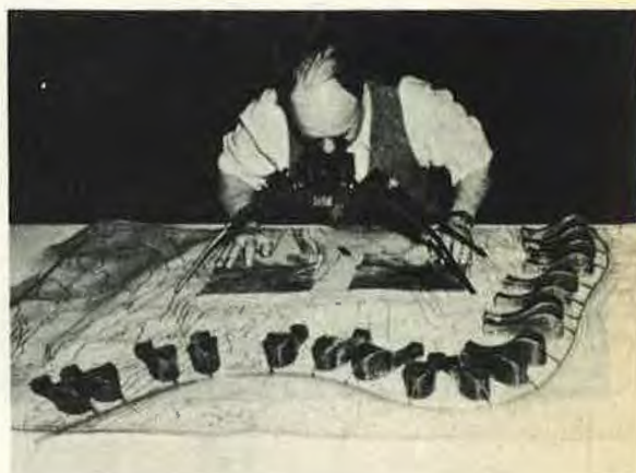
5.—MAKING THE PRELIMINARY SURVEY BY CORRELATING THE PHOTOGRAPHS WITH THE TOPOGRAPHIC MAP
