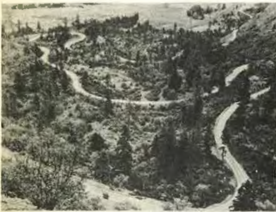
3.- SECONDARY ROAD THROUGH MOUNTAINOUS TERRAIN
