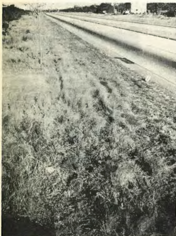
Figure 7. At 3-ft. Offset from Pavement at location 1 (see cut), dry density = 120.2 pcf., voids = 26.7%, organic material = 2.2%, 12.5% passing 200 mesh sieve, turf in good condition in fall of 1947
