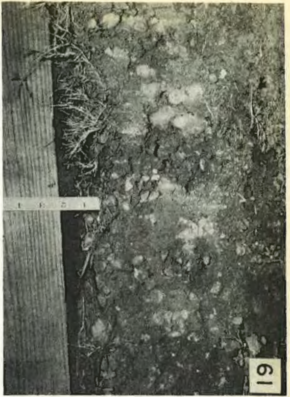
TRAFFIC LANE - 6 INCH CLAY GRAVEL
