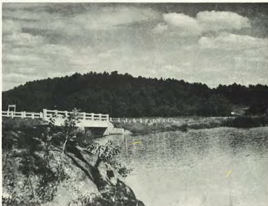
Figure 14. Water resources can be conserved during highway location and construction. Here is a lake covering unsightly mud flats. Note low dam in bridge culvert.
