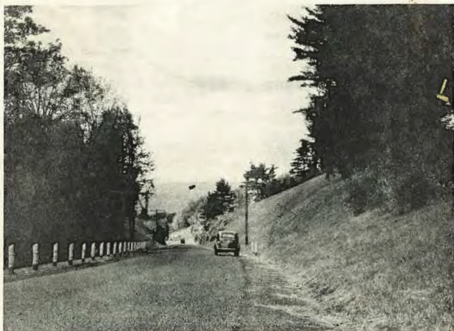
Figure 21. Results of Good Rounded Slope Grading and Mulching and Seeding Immediately Following Construction. Within one year this highway has been completely protected against erosion.
