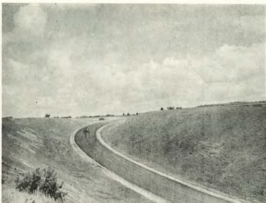
Figure 9. The Same Highway After Reconstruction. Note warped and rounded slopes and clean drainageways. Excellent appearance of this "new" highway is a product not of roadside improvement alone, but mainly of improved cross section design.
