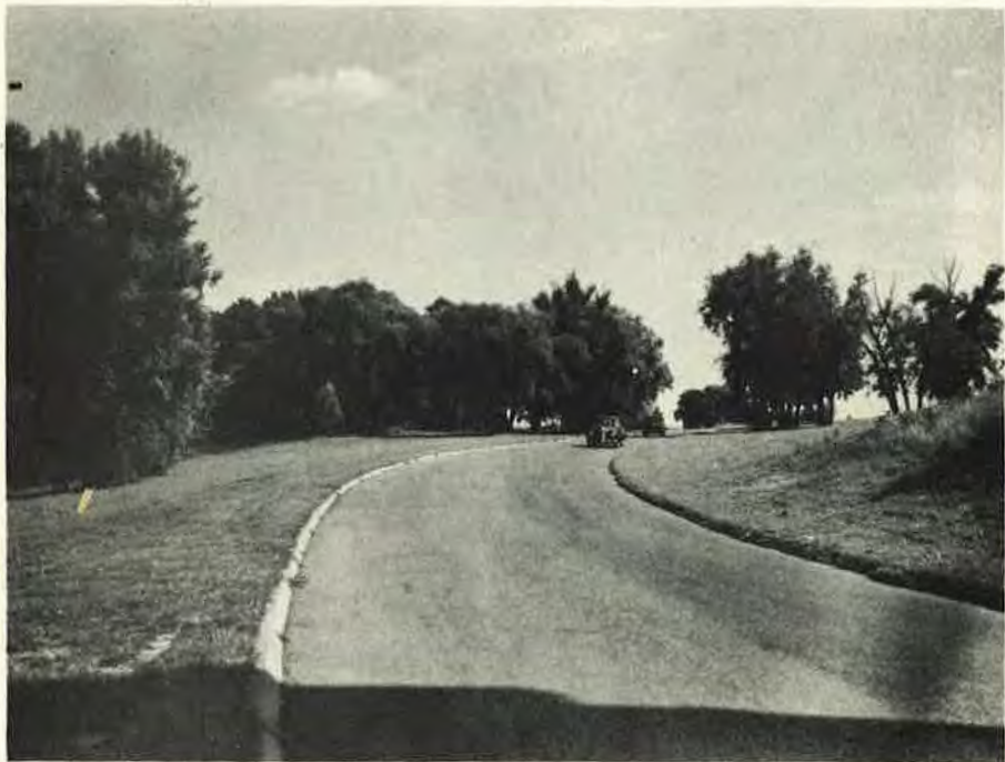
Figure 28. A Section of Controlled Access Highway Where the Essential Requirements of Erosion Control and Tree Planting Were Carefully Considered in Design and Location Stages. Cost of initial roadside development here on an average 300 feet or more of right-of-way about one-third cost of equivalent erosion control work in preceding photograph, per mile of highway.
