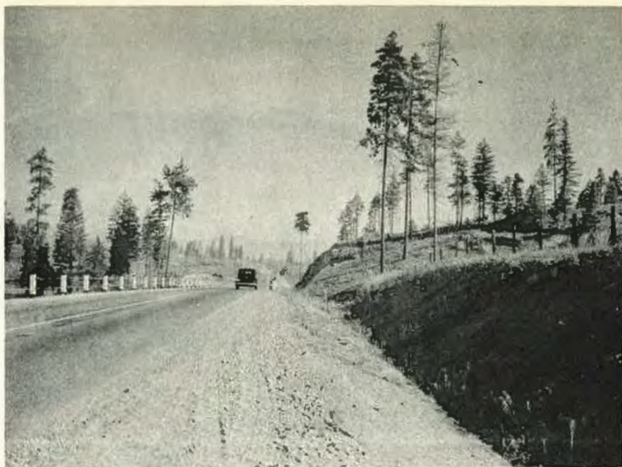
Figure 6. Angular Ditch Cross Section on a Western Highway Constructed In the 1930 Decade. An excellent "man trap"; impossible to protect against erosion.
