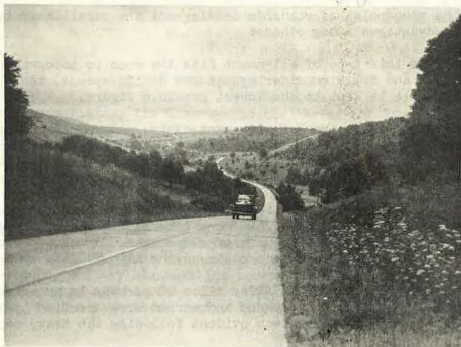
Figure 3. A Highway in Hill Topography With Long Easy Curves Designed to Fit the Lay of the Land. Flowing alignment results in reduced cut and fill and corresponding reduction in roadside development and maintenance costs.
