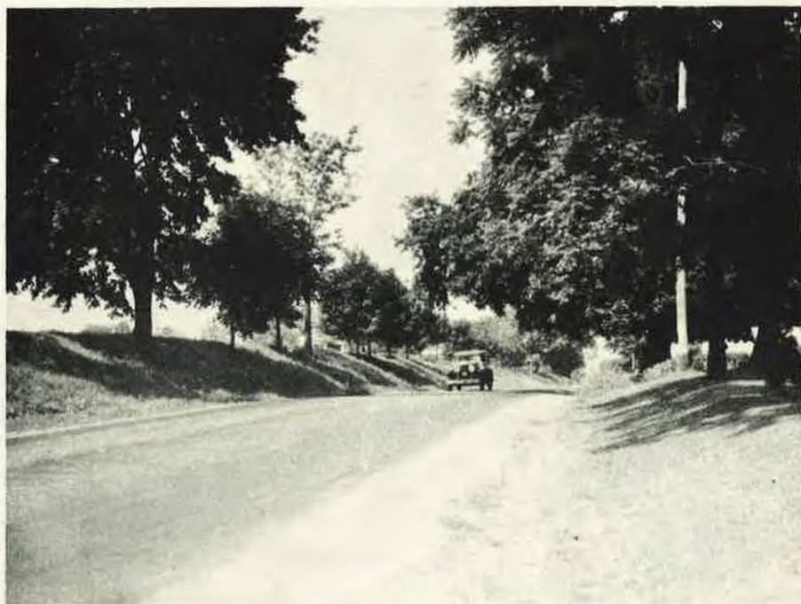
Figure 7. An Improved Modern Rounded Gutter Section, Safe and Easy to Protect Against Erosion.
