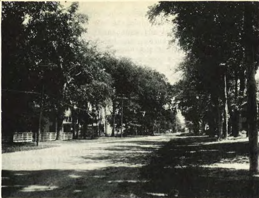
Figure 1. A Highway Right-of-Way More Than a Century Old, With Its Fine Old Trees. This highway is a permanent feature of a New England town. Adequate right-of-way is the first essential for complete and permanent highways.
