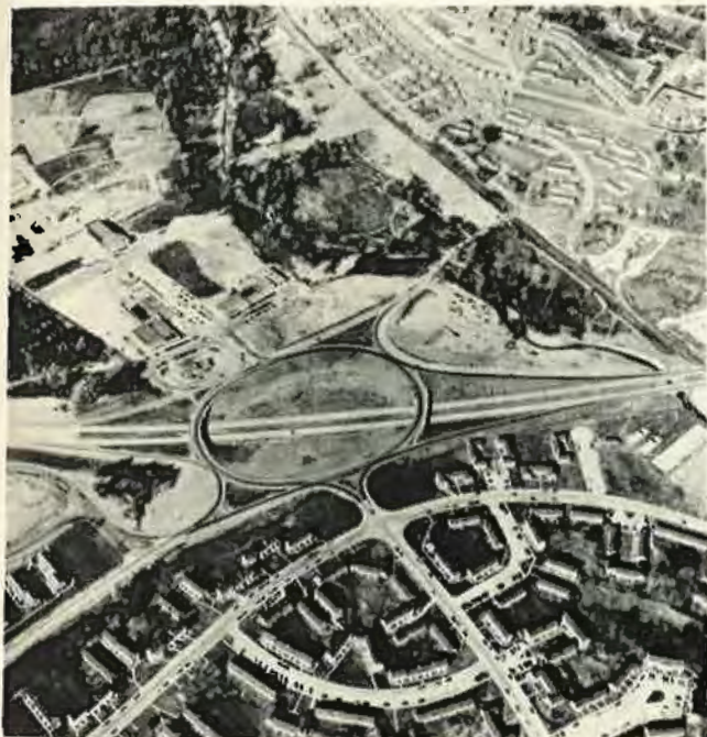
Figure 17. Aerial Photograph of a Grade Separation on a New Controlled Access Highway. A city is growing up in this area which before highway construction was covered by woodland. Increased surface run-off resulting from change in land use has resulted in heavy erosion damage to stream channels and highway gutters.
