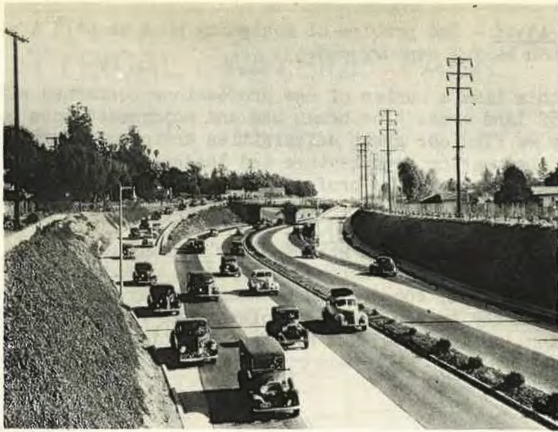
Figure 27. A Section of Controlled Access Highway Where the Essential Requirements of Erosion Control and Tree Planting Were Not Considered in Highway Location, Cross Section Design and Right-of-Way Acquisition Stages. Average costs of erosion control on less than 200 feet of right-of-way were very high per mile of highway on these steep slopes.
