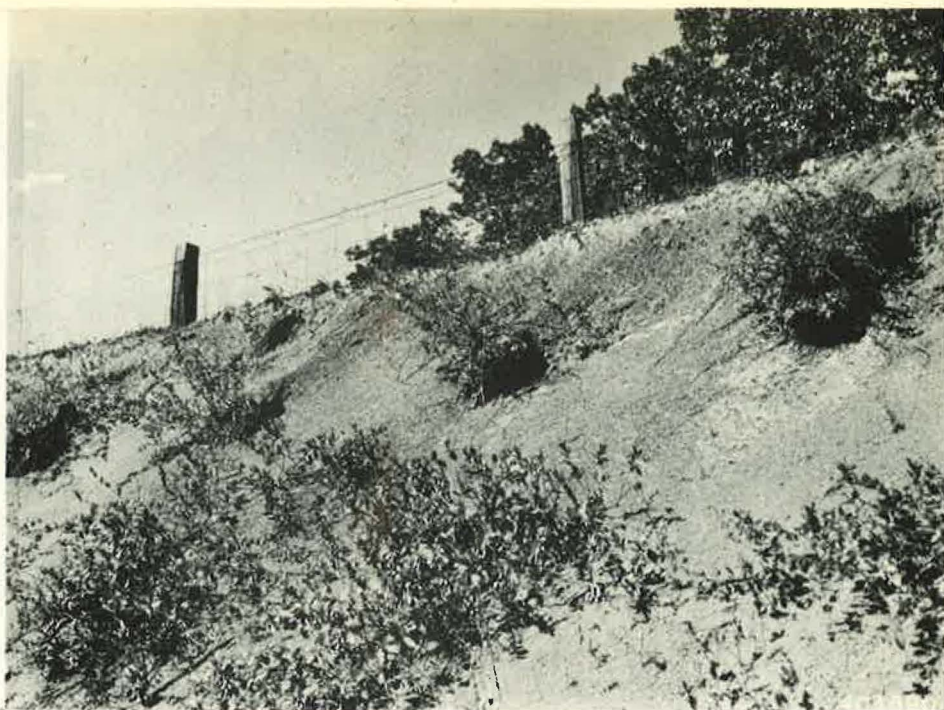
Figure 3. Sloughing due to frost action will remove as much as one foot of bank in a single season. Here the bank has eroded completely away from the large honeysuckle root clumps that were planted in deep pot holes two years earlier.
