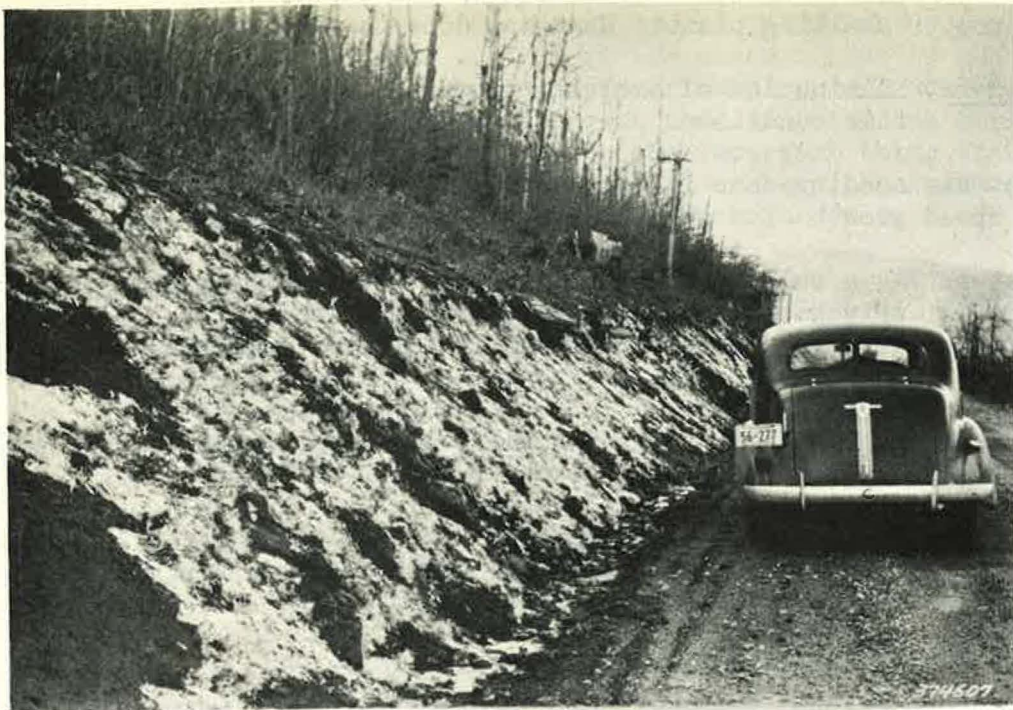
Figure 1. The insulating value of vegetation is well illustrated by the appearance of frost crystals on this roadbank and the complete absence of crystals above the bank.
