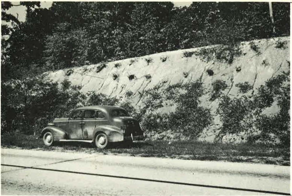
Figure 5. It is difficult to establish vegetation on slopes like this facing toward the south or west. Mulching this slope between the planted vines would have resulted in better and more rapid growth.
