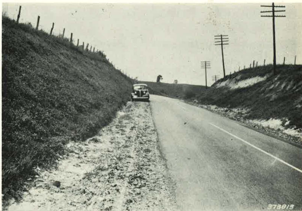
Figure 4. Recognition of difficult planting sites is important. The south facing slope to right will require many times the amount of effort to achieve vegetation establishment as a north facing slope on the left. Both banks were planted in the same manner.
