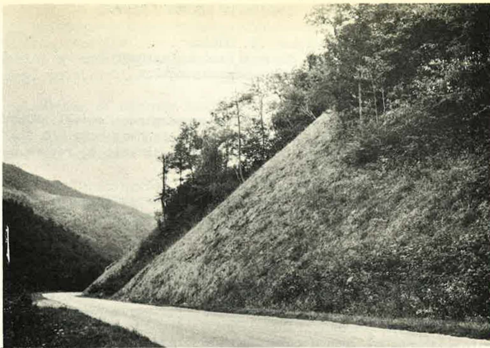
Figure 11. Blending steep slopes into the landscape presents some difficult mulching and planting problems, but the job can be done. This slope was bare a few years before the photograph was taken.
