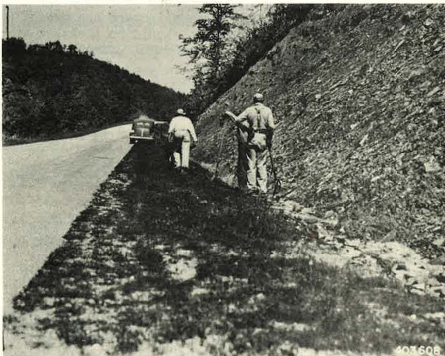
Figure 12. A cover of mulch, and seeded or planted ground cover would have saved money in maintenance here. The shoulder was seeded but erosion on the cut slope requires cleaning out of ditches after every storm, and after the frost action of every winter.
