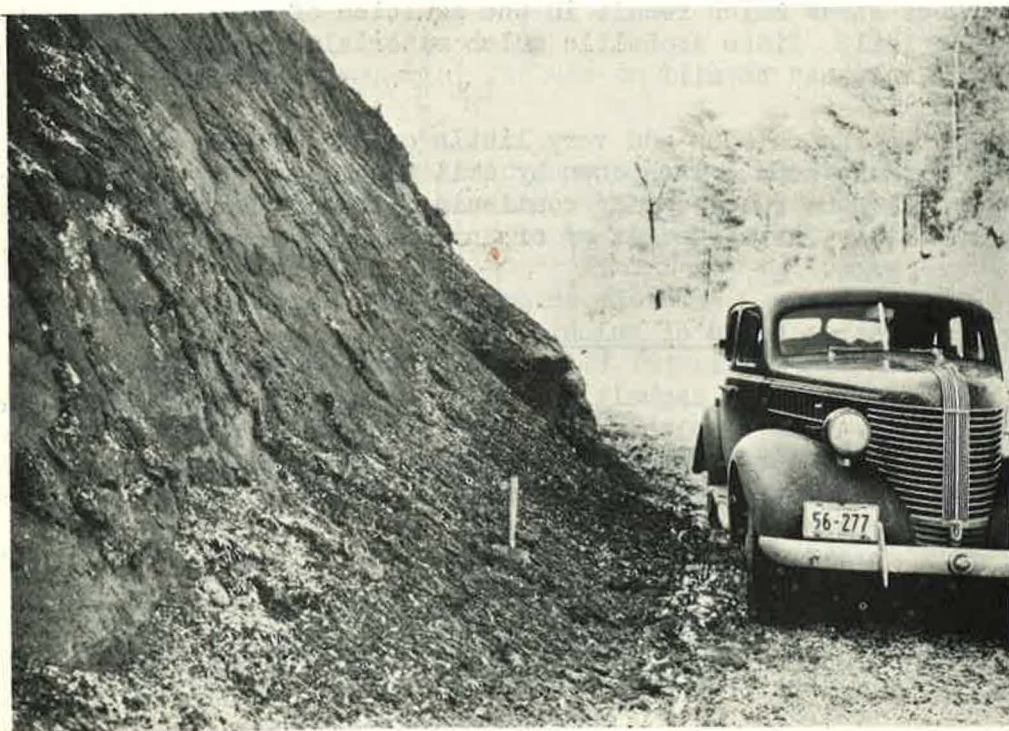
Figure 2. Alternate freezing and thawing may take place more than 50 times in a single winter season within the frost belt of the United States. Note loose material dislodged by frost action lying at foot of this cut slope.
