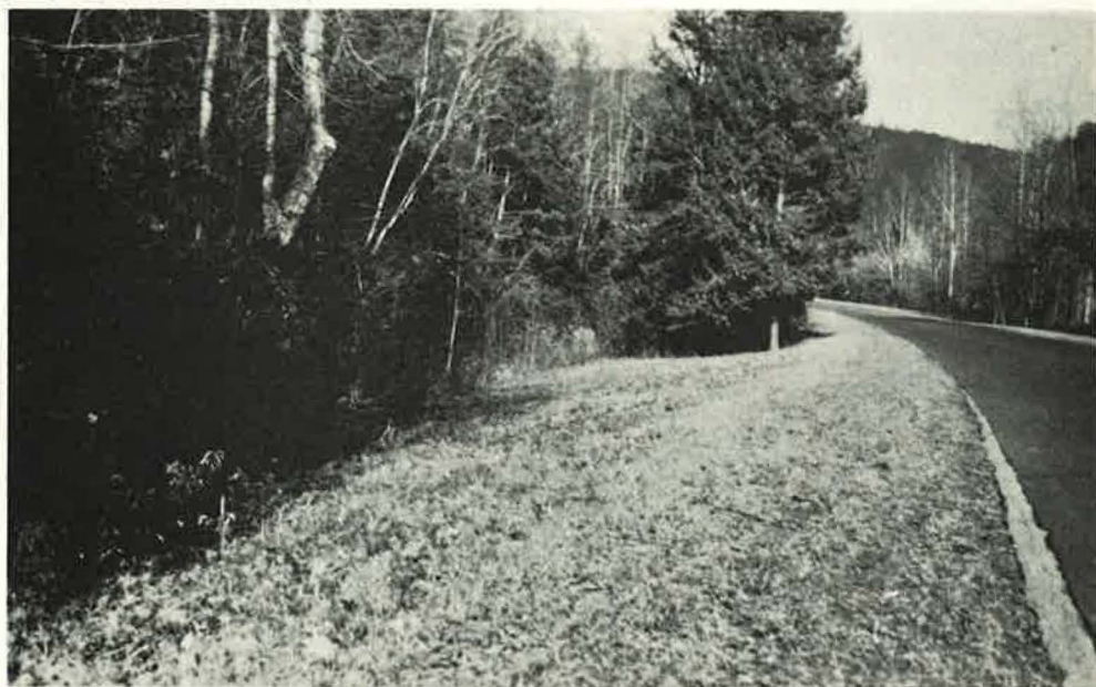
Figure 10. Moderate-Sized Pocket Fill Built on 10 to 1 Slope From Shoulder. Tree in Background was Carefully Preserved During Construction Operations. Such Pockets are Convenient Places to Dispose of Surplus Excavation.
