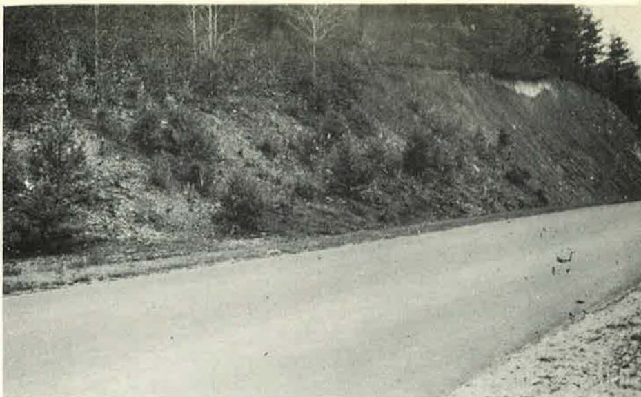
Figure 1. In Moist Climaté of the Great Smoky Mountains National Park Volunteer Vegetation will Grow on Slopes of 1\frac{1}{2} to 1 or Flatter (center) but Ravelling Removes Seedlings from 1 to 1 and Steeper Slopes (right). Ravelling is very Active Due to Numerous Cycles of Freezing and Thawing. This slope is 12 years old.
