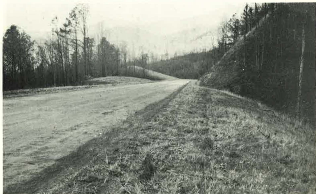
Figure 6. Variety Can Be Imparted to the Roadside by Varying the Slopes of Residual Hillocks. Such Treatment Also Provides Flexible Source of Borrow.
