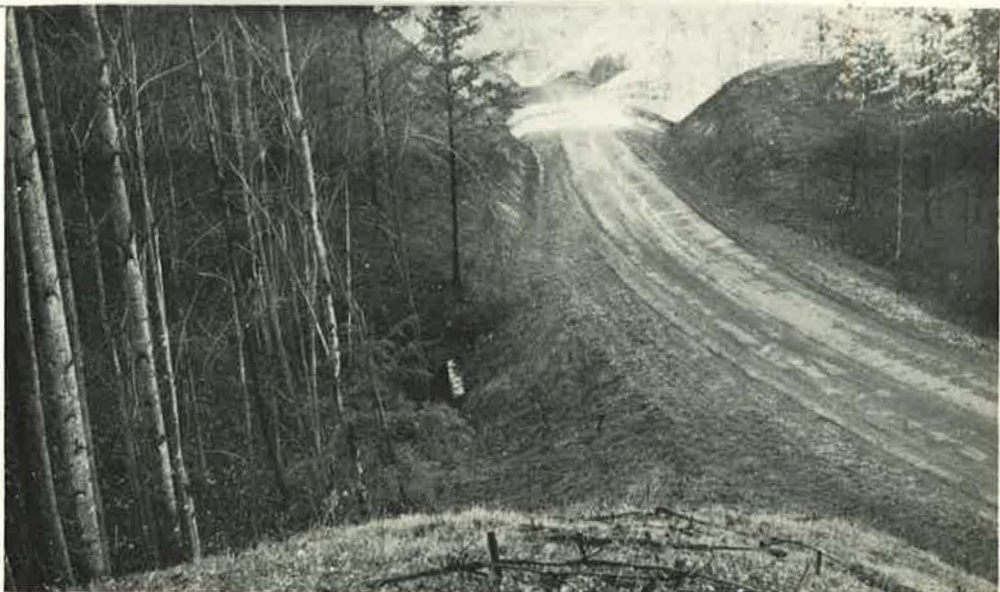
Figure 14. Bell-Mouthing of Cuts, Combined With Rounding and Transitioning Produces Natural Basic Ground Shape. Gutter at Exit of Cut in Foreground is Wide and Shallow to Reduce Erosion. Rounding is Clearly Evident on Dark Silhouette of Cut in Middle Distance.
