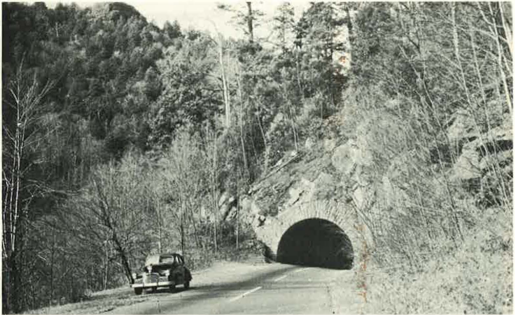
Figure 12. Severe Damage to the Landscape Can Sometimes be Avoided at Little Extra Cost by Tunnelling.
