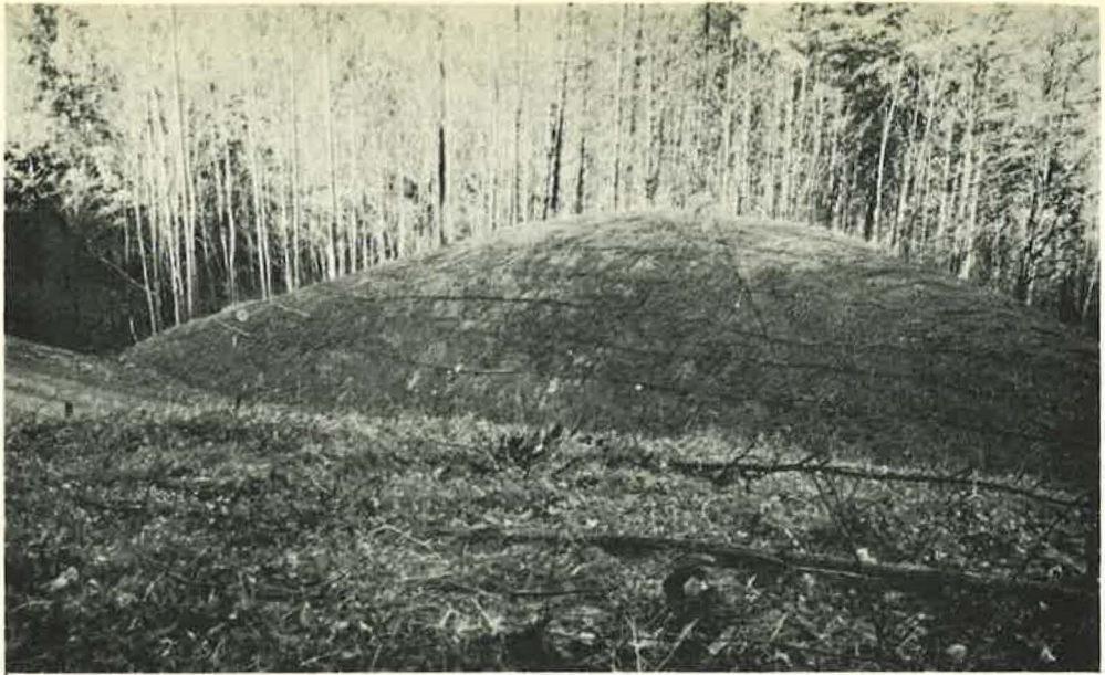
Figure 15. Graded Surfaces are Seeded and Mulched. Mulch is Held Down by Saplings Obtained by Thinning Adjacent Forest.
