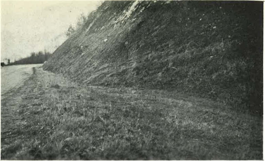
Figure 19. Bell-Mouthed and Rounded Transition Supports Luxurious Growth of Vegetation Five Months After Completion of Grading. Shale Slope in Background is on 1 to 1 Slope and Was Not Seeded.
