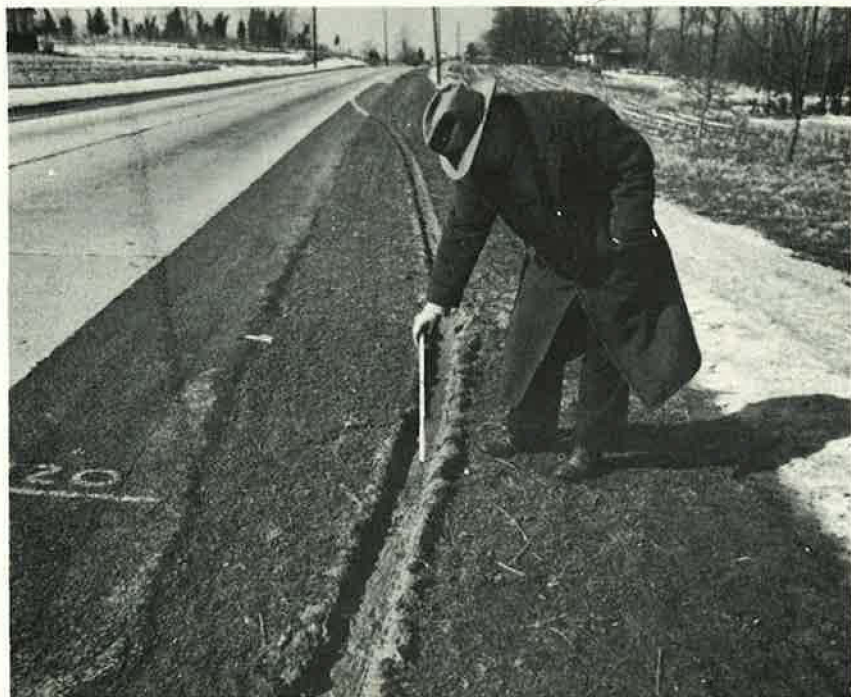
Figure 3. Rutted Turf Shoulder After Period of Thawing. Rut 1''-1\frac{1}{2}'' deep. Feb. 19, 1948.
