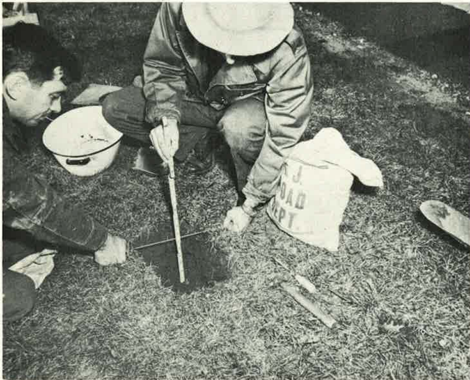
Figure 9. Sample Test Hole Station 217709. Depth of Top Course .65 Ft. November 15, 1948.
