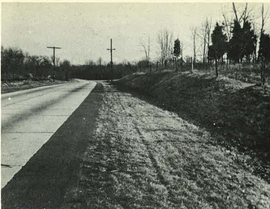
Figure 12. Stabilized Turf Shoulder Cover With a Dense, Tough, Growth of Vigorous Grass. Station 213/0. November 15, 1948.
