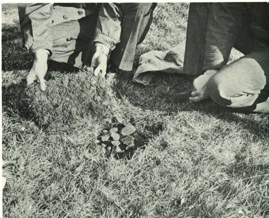
Figure 7. Removing Sod and Stone Aggregate From Test Hole - Station 213/71 R. Nov. 15, 1948.
