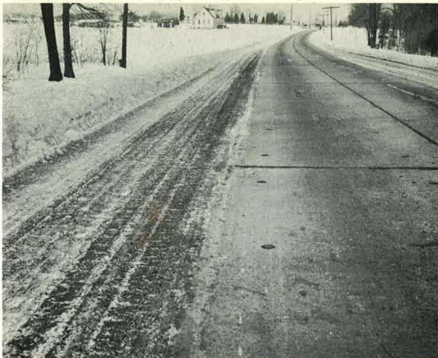
Figure 2. Wheel Tracks Indicated that Considerable Traffic Had Used Shoulder. Jan. 27, 1948.
