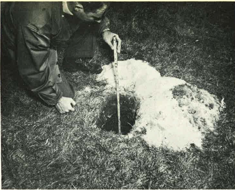
Figure 8. Test Hole Station 21370 - Total Depth of Stabilized Materials 1.20'. Nov. 15, 1948.
