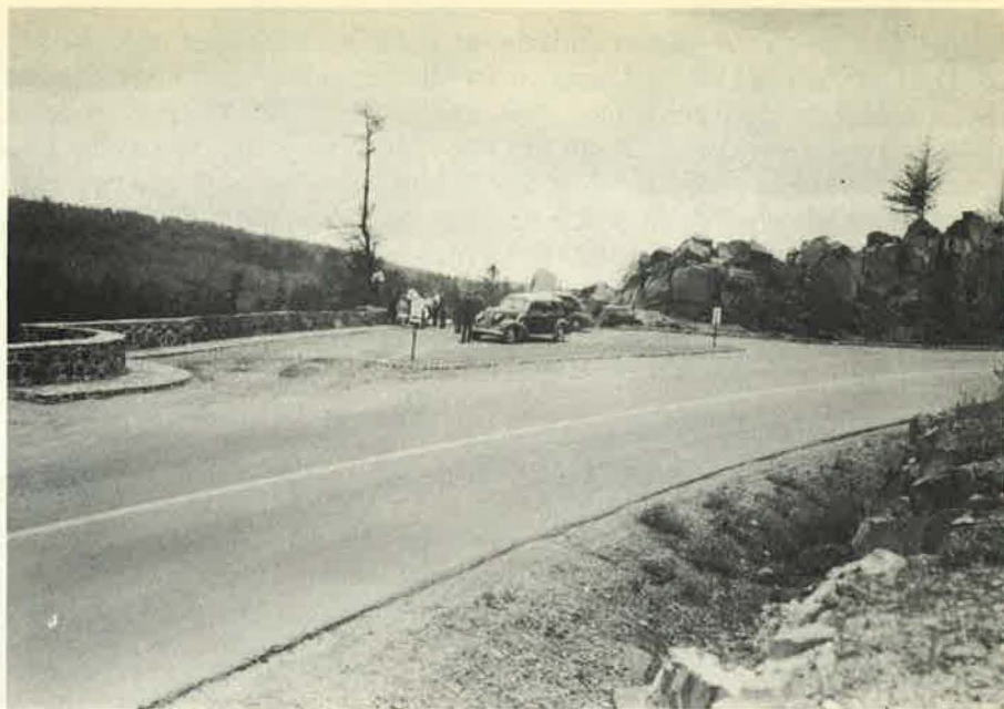
Figure 12. Scenic turnout on a Minnesota Trunk Route in the Interior Plains region. Note island separation and masonry curbs and sidewalk. This area will not be readily damaged by heavy use.
