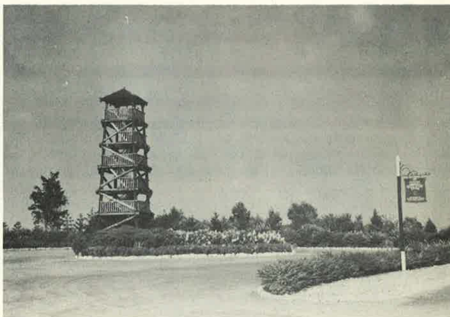
Figure 21. Early type of wayside rest area, northeastern Appalachian Highlands region. Log structures of this type are subject to decay, and are a hazardous feature not usually to be recommended for roadside installation.
