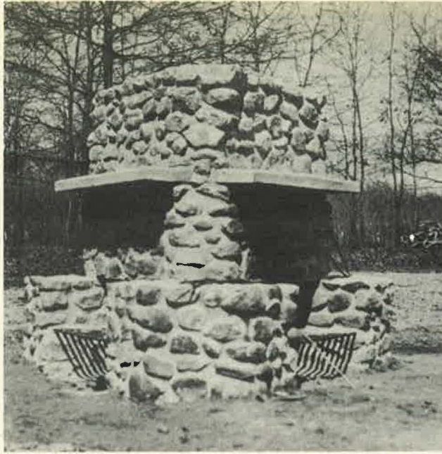
Figure 26. A roadside fireplace, costly, bordering on the grotesque in appearance, and requiring too much fuel for economical use. Note excessive bulk of chimney and over-large fire compartments, out-of-scale with parklike surroundings.
