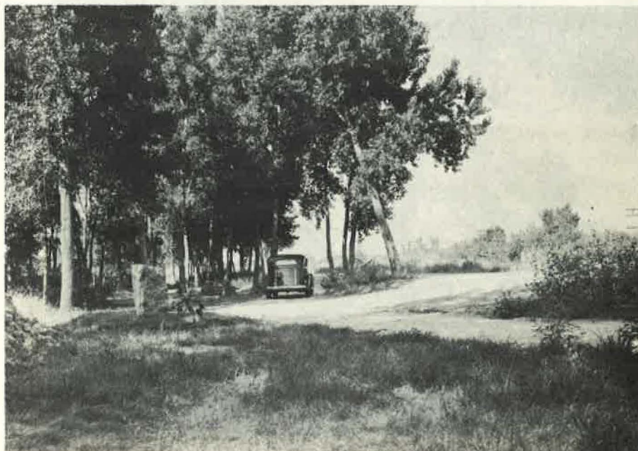
Figure 7. Turnout on a highway in the southern Interior Plains region. Note tables and benches and parking space. Rising grade at exit point to road and apparent lack of sight distance would appear to introduce a traffic hazard here.
