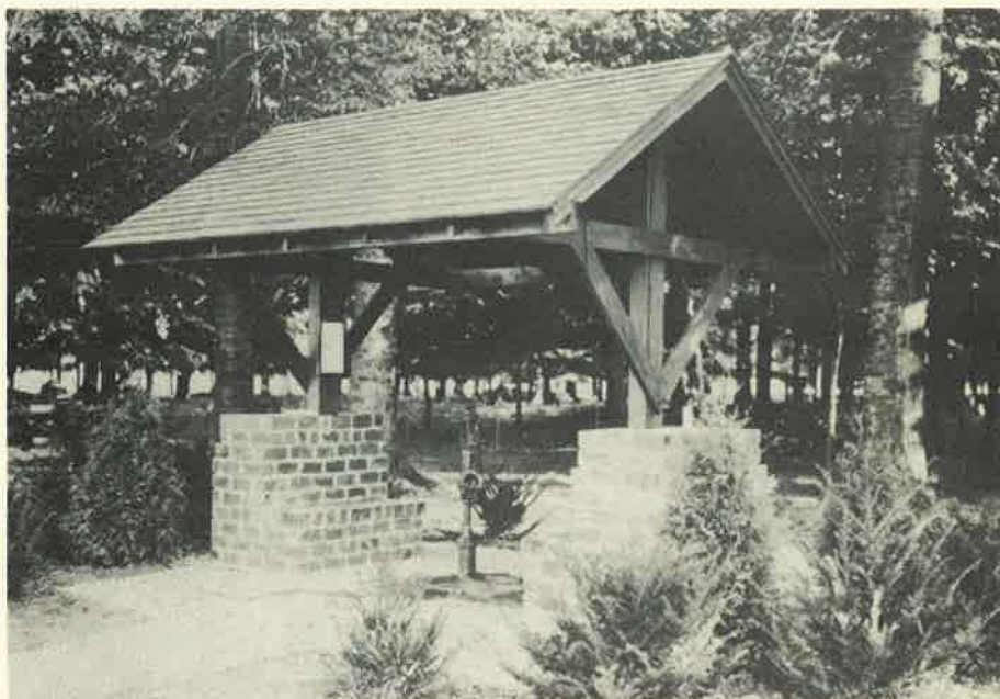
Figure 25. Close-up of typical pump shelter (Ohio).
