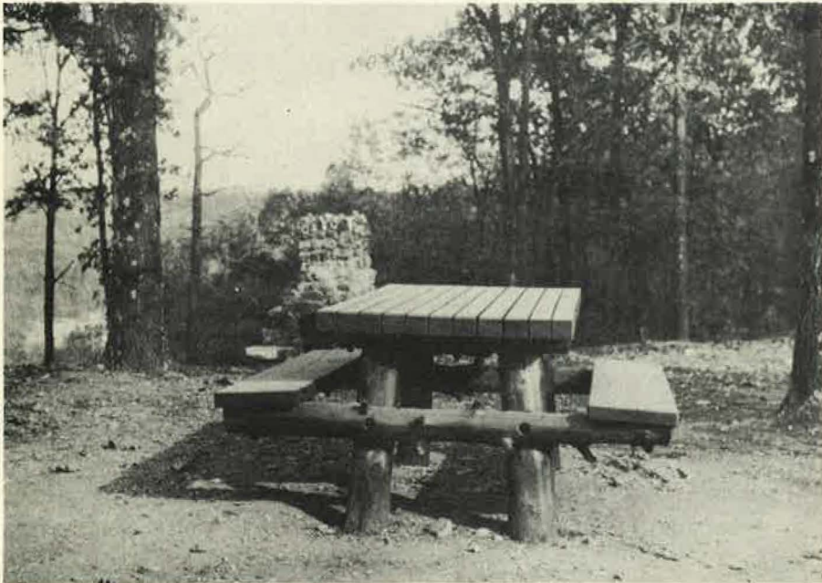
Figure 23. Heavy timber table and bench. Creosoted where it meets the ground. Excellent in design, except for stubs on cross pieces that are a hazard to clothing.
