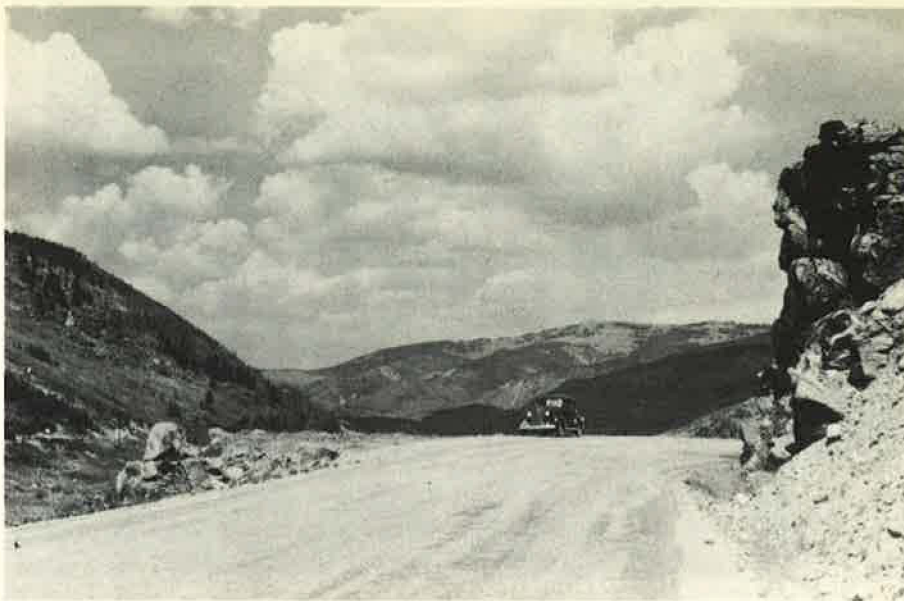
Figure 2. Site for a scenic turnout--Rocky Mountain region. Bumper rails to protect vehicles, and a separating island, will be needed here to make this excellent turnout site safe for public use.
