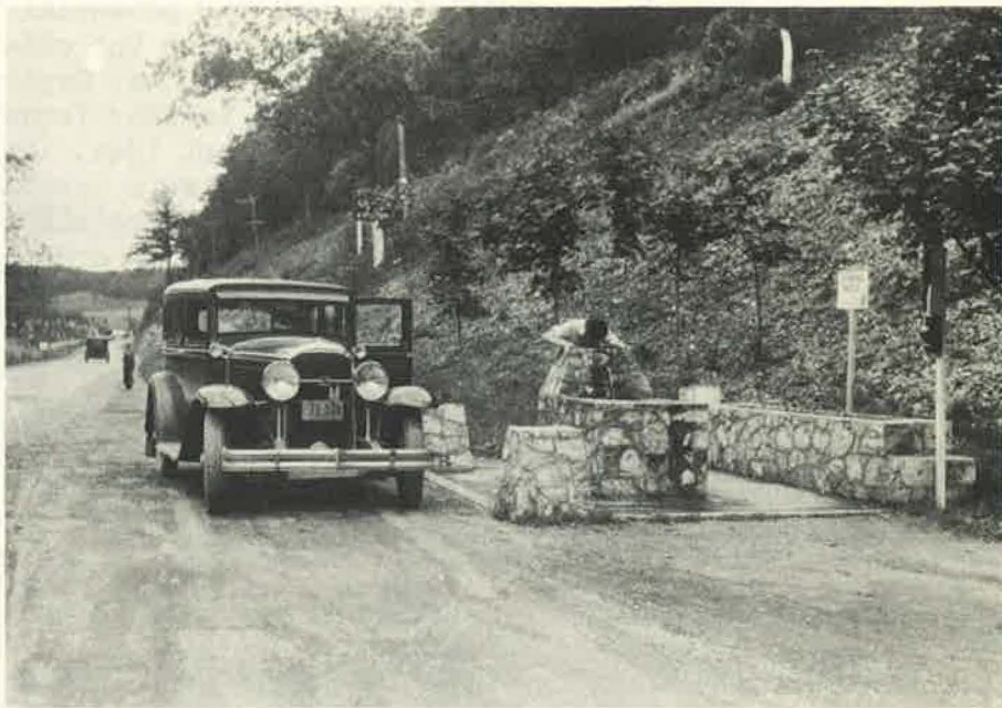
Figure 13. Turnout and drinking fountain, Appalachian Highlands, West Virginia. It has been found difficult to protect roadside springs against contamination. Wells appear to be the safer source of water supply.
