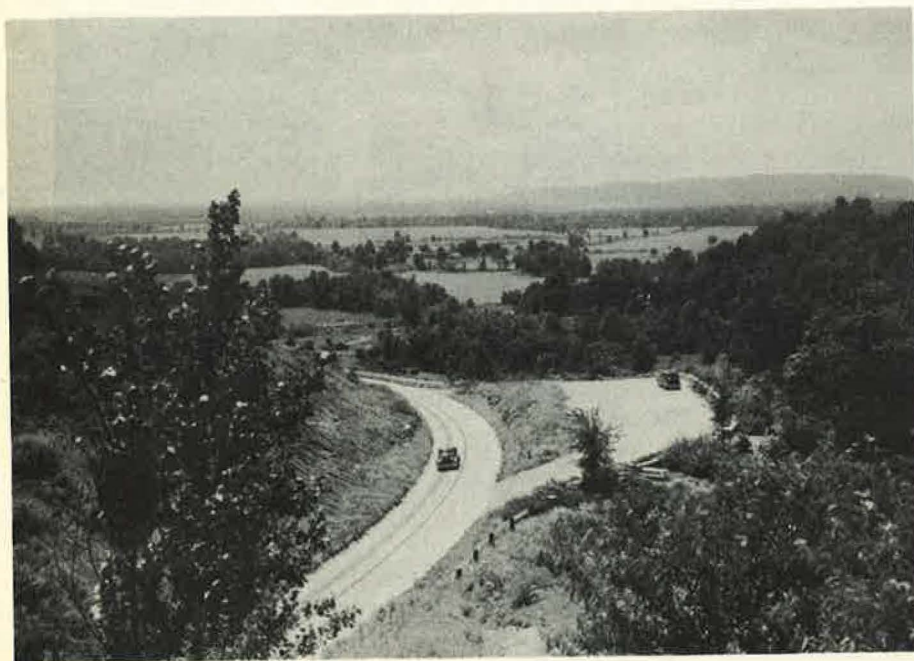
Figure 17. A dangerous turnout area. Note short sight-distance at entrance and exit points, and steep driveway grades.
