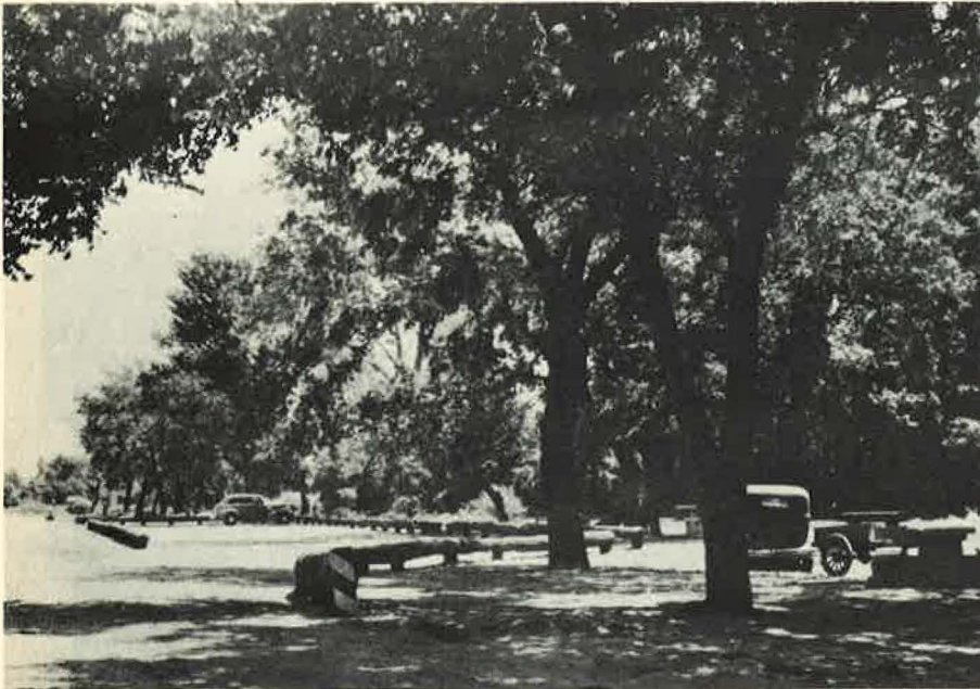
Figure 9. Wayside rest area Interior Highlands region (Missouri). Note facilities provided for parking, and types of table and bench units.
