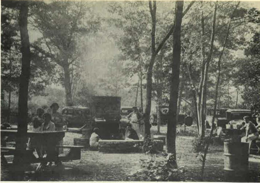
Figure 28. Order in arrangement of driver service facilities is essential. Lack of orderly arrangement is evident here.
