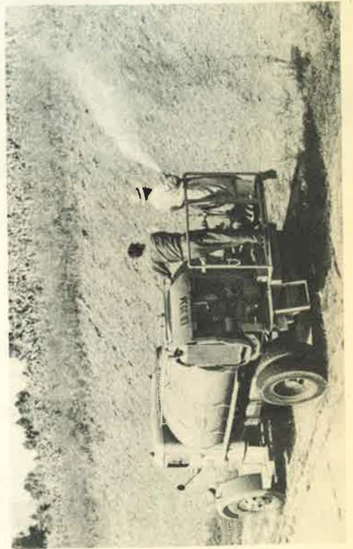
Picture No. 23 - Seed and Fertilizer Sprayer
