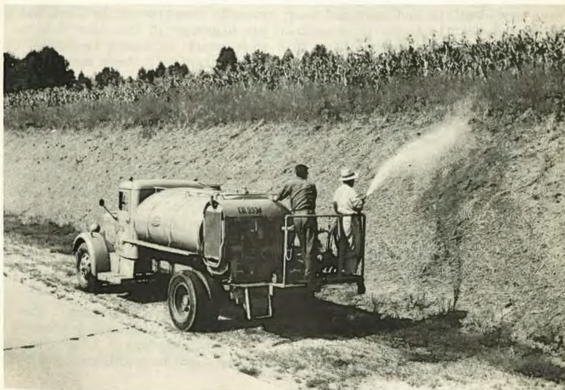
Figure 3. Virginia's Seed and Fertilizer Sprayer is Demonstrated on the Shirley Highway.
