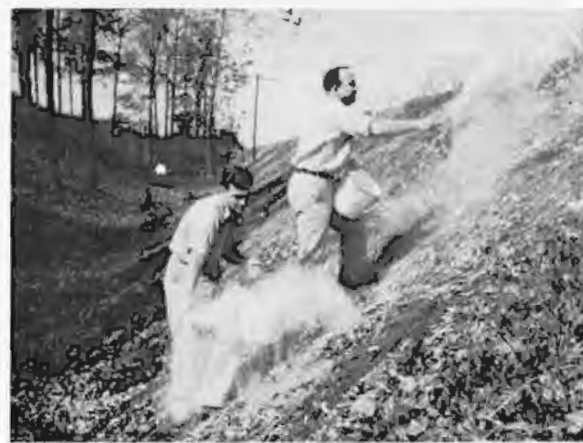
Figure 11. Hand broadcasting the dry resin.
