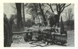
Stone Rake - This machine, which can be towed by truck or tractor, can be adjusted as to height by a hand-operated hydraulic lift. The frame is of steel channel iron. The spring-steel times are bolted between two pieces of steel which hold them in place. The angle of the rake is adjustable by rotating the front of the frame and tongue. Coil springs allow for the release of pressure exerted on the surface when an obstruction is encountered.
