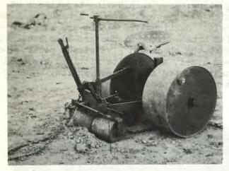
Sod Cutter - This sod cutter is towed by truck, tractor, or jeep. The cutterbar is an arrow-shaped plow which cuts onehalf a strip of sod at a time on each side of the rolling coulter wheel. The depth of cut is regulated by a hand lever. The machine is steered by means of a handle bar so that the sod can be cut to a line by using a guide arm at the front of the machine. The rear wheels may be filled with gravel or water if desired.
