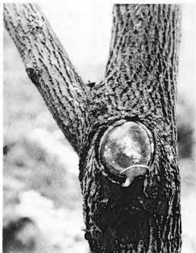
Figure 7. This unpainted cut became infected by a wound parasite which causes heart rot. A fruiting body of this fungus appears at the base of the scar.
