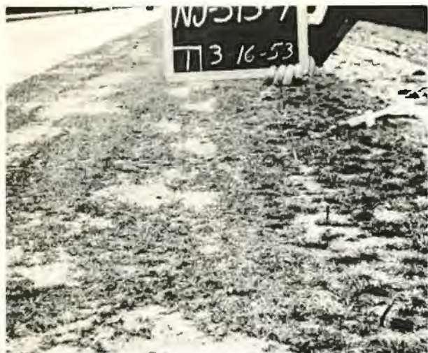
Fig. 2. Test Area NJ-STS-7 prior to traffic test.
