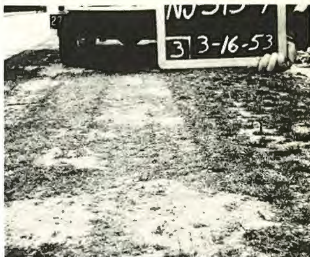
Fig. 3. Test Area NJ-STS-7 after four passes of loaded truck.
