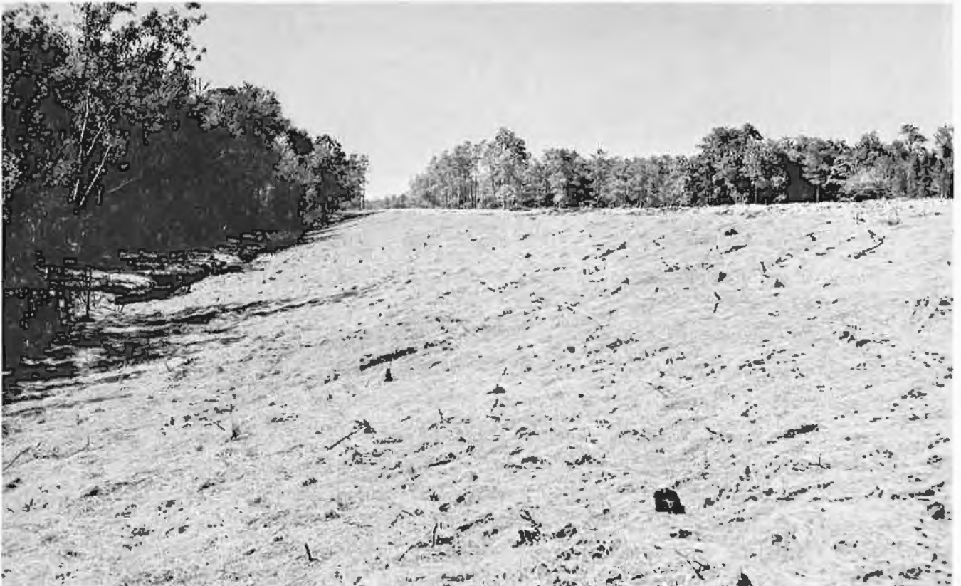
Figure 4. Peat from storage piles (see Figure 3) was disked into the surface of the sand fill which was then limed, fertilized, seeded, and mulched.
