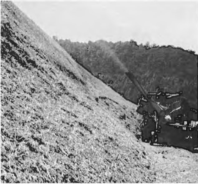
Figure 2. The idea of spreading the straw and tying it to the soil with asphalt emulsion in a single operation greatly speeded up operations.
