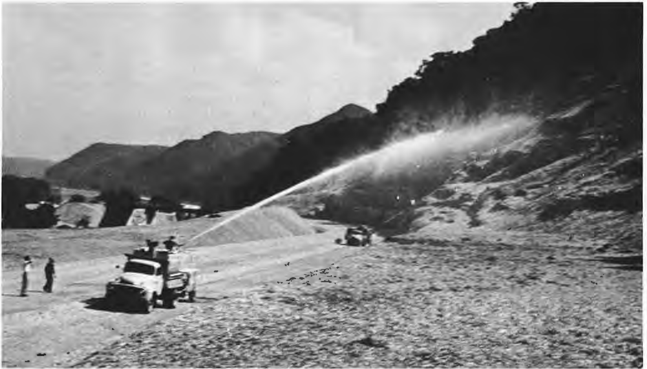
Figure 3. An output of 100 gal. of seed and fertilizer mixture per minute and a distance of 125 feet were possible with the hydraulic seeders used on the West Virginia Turnpike.
