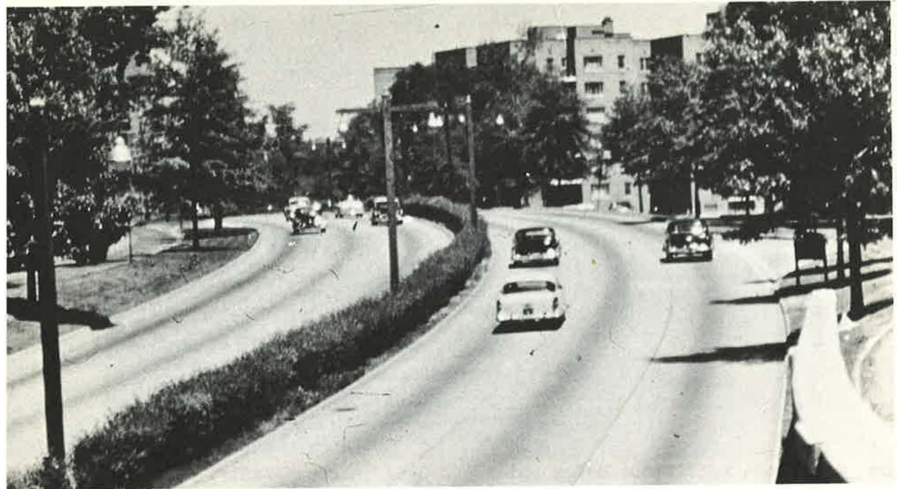
Figure 5. Crataegus crusgalli (cockspur thorn) hedge in a narrow median on the Henry Hudson Parkway, Riverdale, N. Y., makes an effective headlight-glare screen and delineator of changing alignment.
