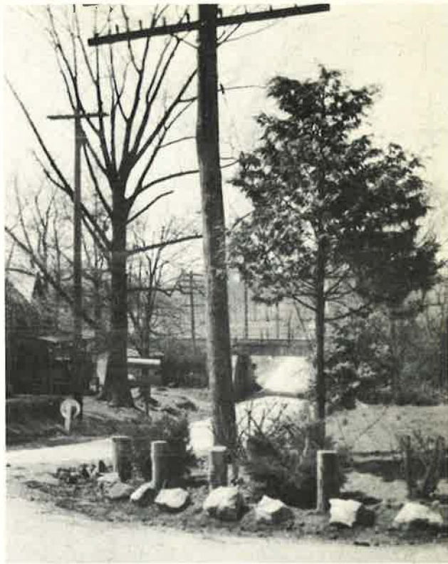
Figure 3. Before (left) and after (right) selective removal of vegetation to improve sight distance at rural intersection. (Maryland State Roads Commission.)
