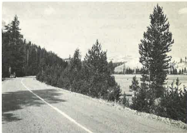
Figure 5. Young pines on fill slope on curve are reducing sight distance and closing vista of meadow.
