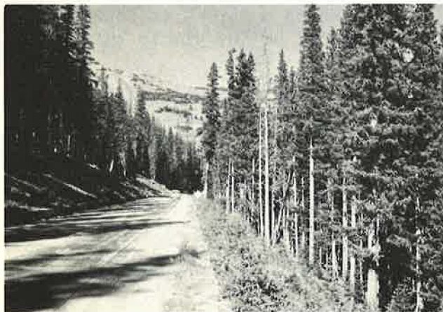
Figure 4. Dense growth of young evergreen trees on fill slope will eventually require thinning.
