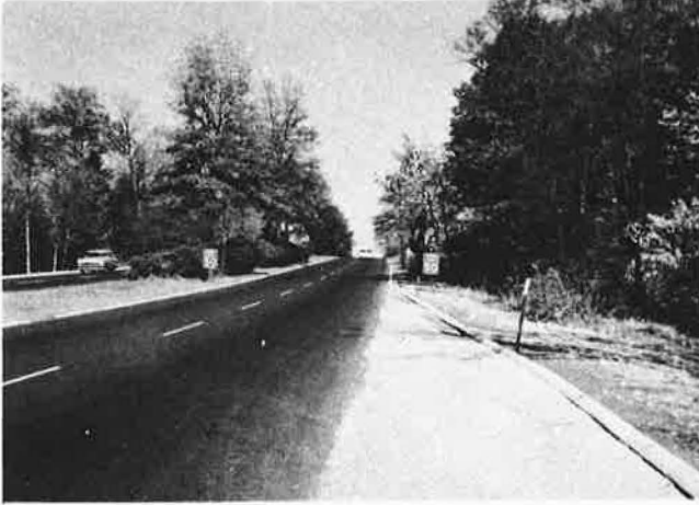
Figure 6. Planting for screening headlight glare, consisting of mountain laurel, flowering dogwoods, and pin oaks, on the Merritt Parkway in Connecticut. Underplanting of mountain laurel produces an excellent year-round evergreen screen. (Photo by Charles Brennen)
