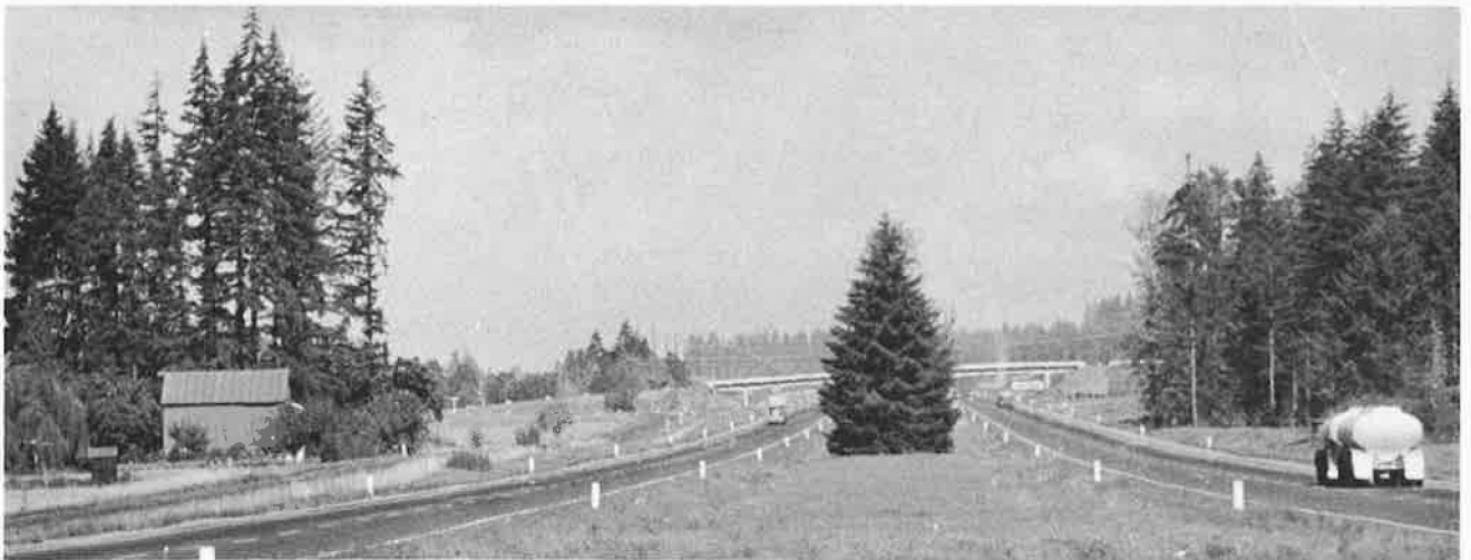
Figure 13. A view of the R. H. Baldock Freeway in Oregon, showing the value of a single Douglas fir tree ( Pseudotsuga taxifolia ) in the median. Opposing traffic lanes are 100 feet apart. (Courtesy Oregon State Highway Department)
