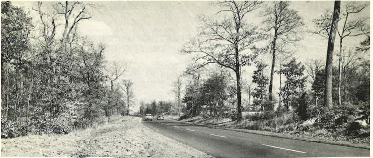
Figure 2. Varying width of median on the Palisades Interstate Parkway allows native woodland growth to remain undisturbed between opposing roadways. (Courtesy New Jersey State Highway Department)
