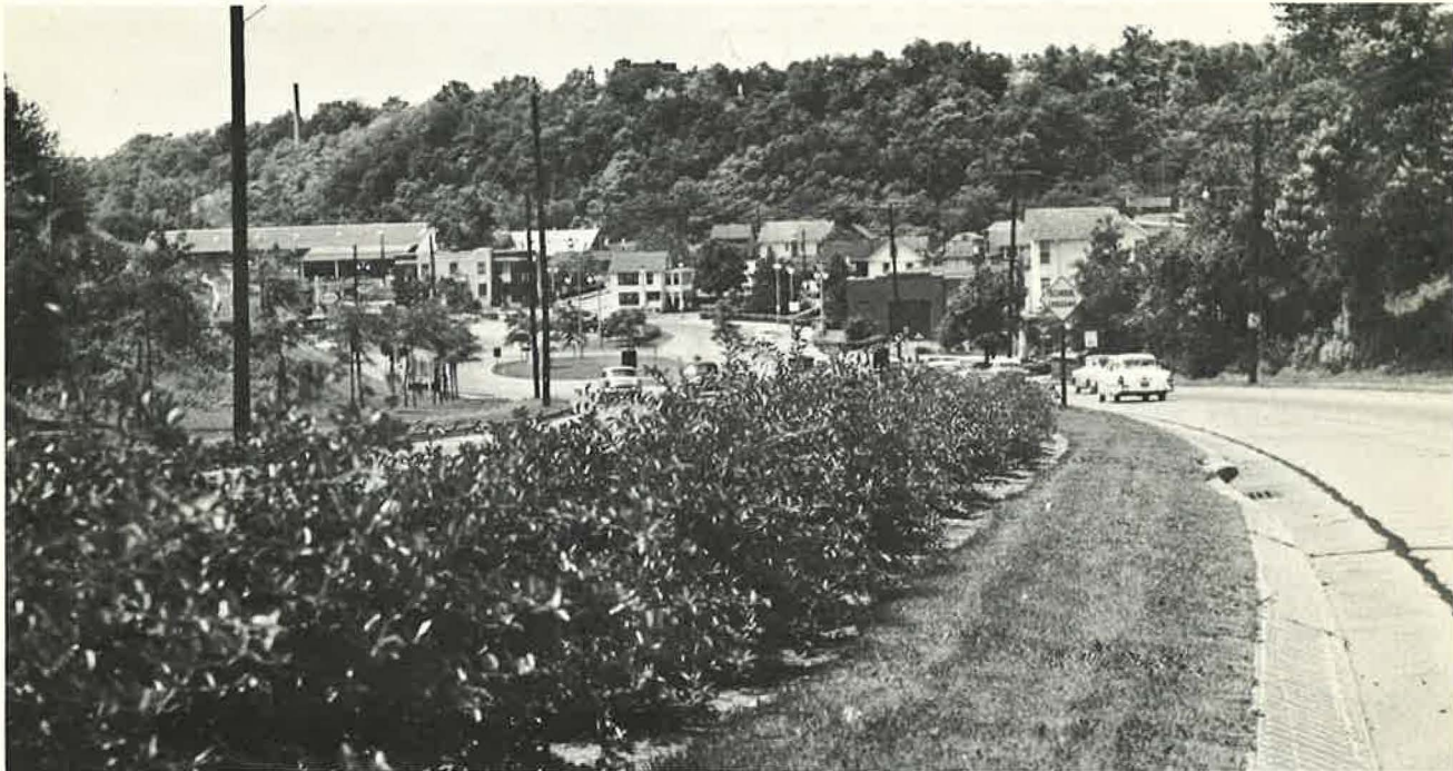
Figure 10. On US 22, Phillipsburg, Crataegus crusgalli screen planting for headlight glare and traffic guidance, looking toward the Delaware Bridge Plaza. Median measures 15 feet. (Courtesy New Jersey State Highway Department)
