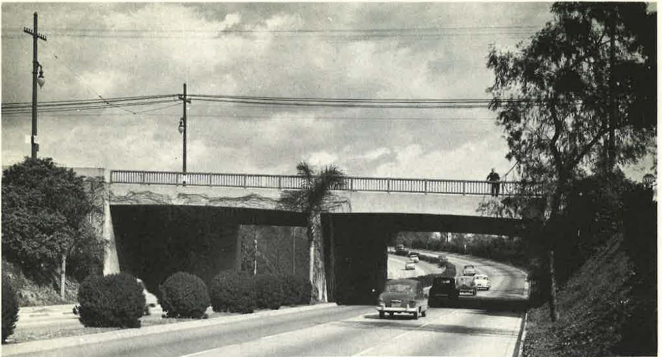
Figure 4. Arecastrum romanzoffianum and Eucalyptus sideroxylon rosea planted at bridge piers and abutments of the Fair Oaks Avenue Bridge, Pasadena Freeway, to emphasize the restricted roadway. (Courtesy Division of Highways, California Department of Highways)
