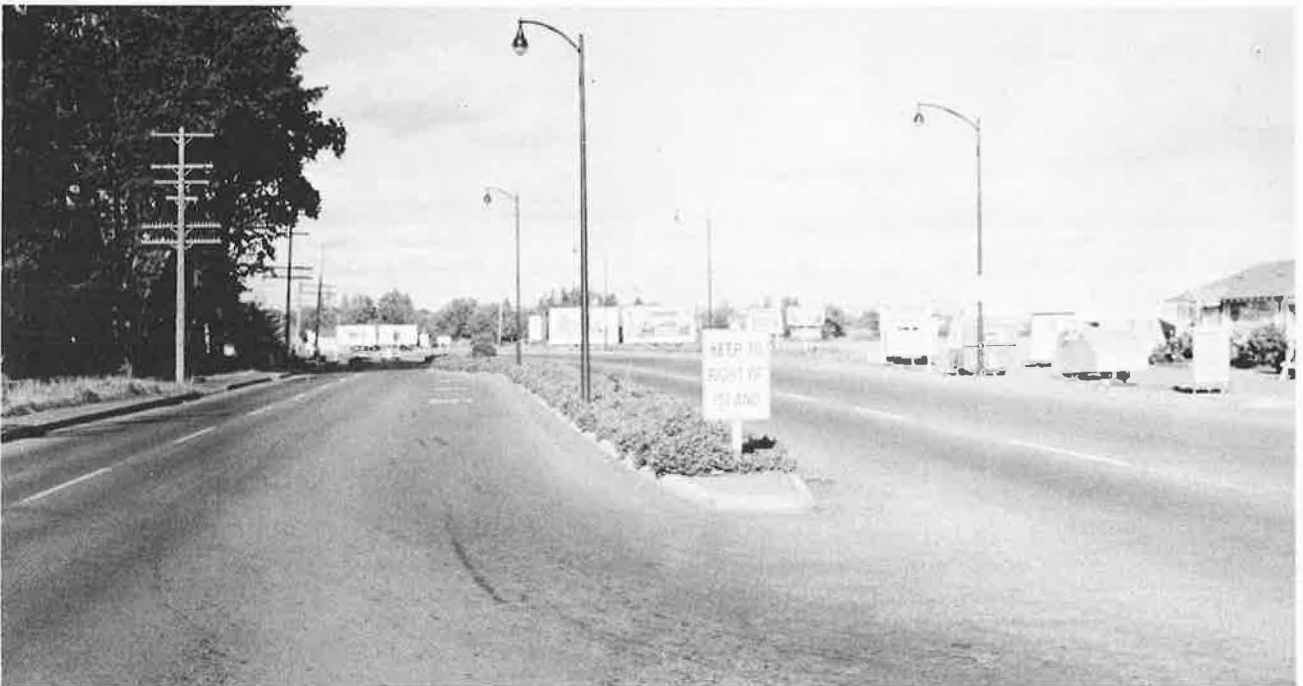
Figure 15. A planting of salal ( Gaultheria shallon ) in a median at McMinnville, Ore. This evergreen plant has served admirably to accent the island without interfering with sight distance at this intersection. The plant has an added virtue; it can be mowed with sickle-bar mowers and retained at any height desired. (Courtesy Oregon State Highway Department)
