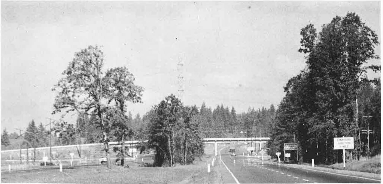
Figure 14. A view of the R. H. Baldock Freeway between Salem and Portland, Ore. These natural groupings of Oregon white oak ( Quercus garryana ) were retained in the median and between the frontage road and the main highway. The opposing lanes are 100 feet apart. (Courtesy Oregon State Highway Department)
