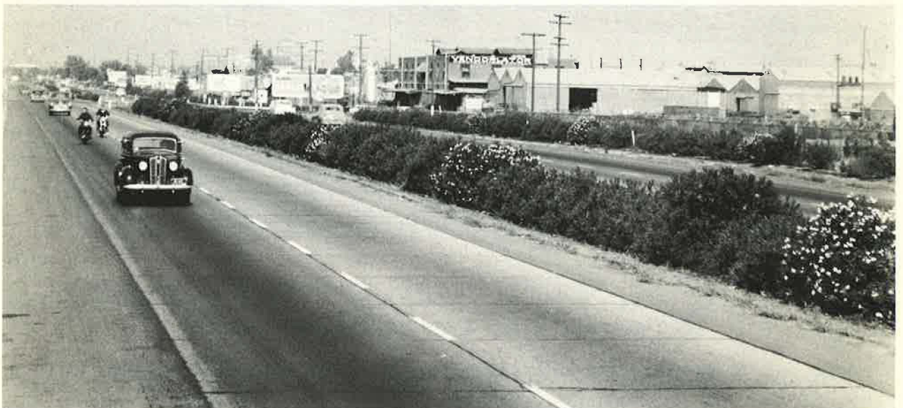
Figure 3. Nerium oleander in median and along right-of-way on California 4B, Fresno. (Courtesy Division of Highways, California Department of Public Works)
