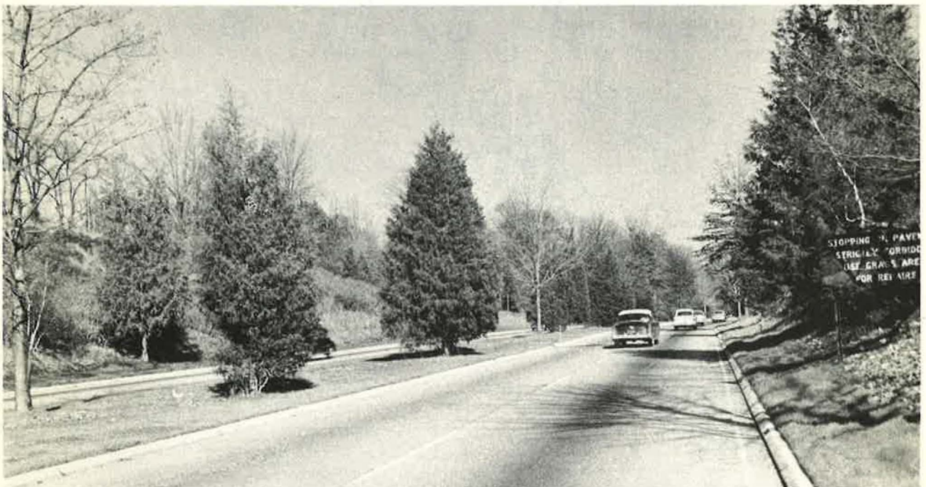
Figure 5. Effective red cedar and sugar maple planting in 20-foot median on the Merritt Parkway, Connecticut. (Photo by Charles Brennen)
