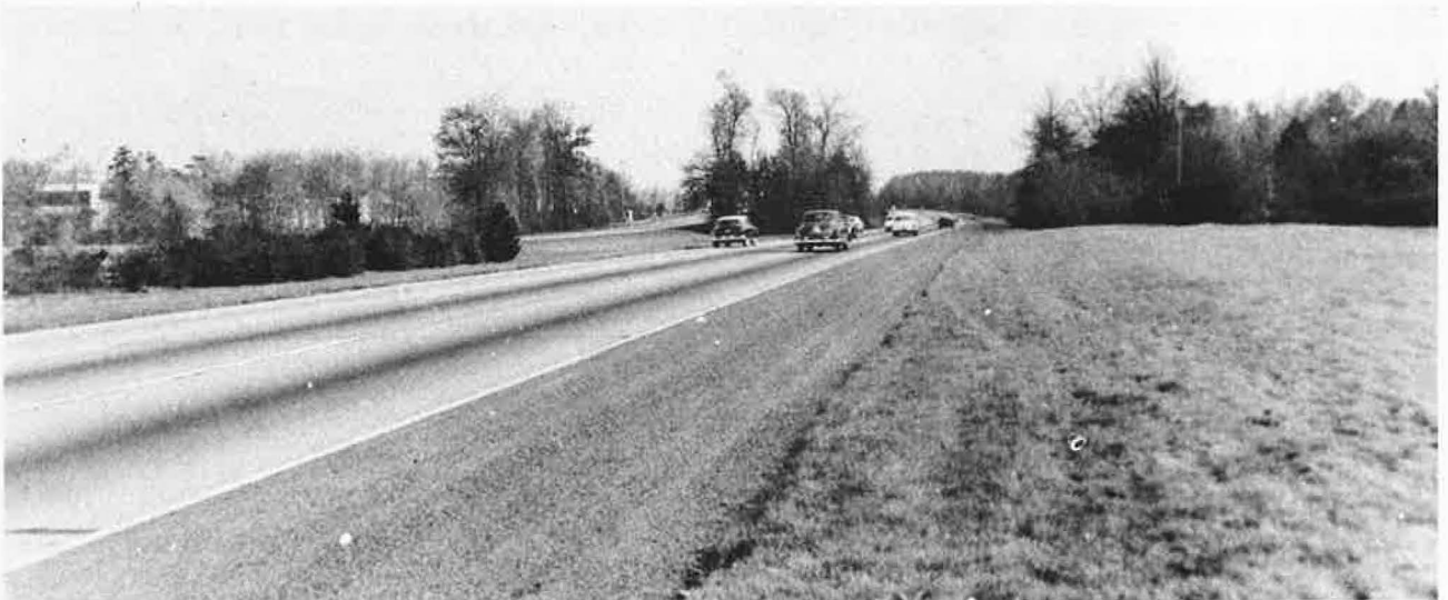
Figure 1. Acquisition of wide right-of-way permits a more flexible location of the roadways and adjustment of the profiles so that large areas of native trees and shrubs may be conserved as a headlight-glare screen. View of Garden State Parkway. (Courtesy New Jersey State Highway Department)
