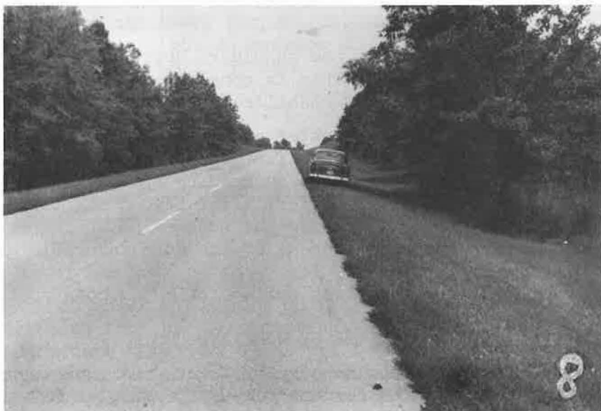
Figure 11. Good cover of turf on stabilized shoulders of the LJ2 portion after three full growing seasons.
