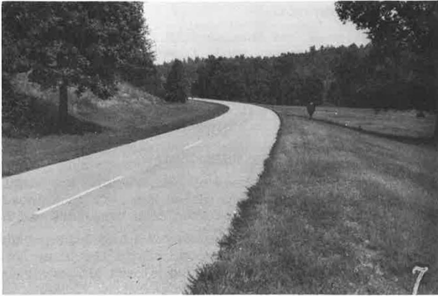
Figure 10. Typical for the 12-mile LH6 portion (Tennessee) after three full growing seasons. Lush growth might subside upon discontinuation of yearly booster application of fertilizer.
