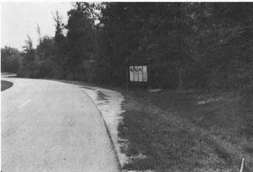
Figure 9. See general comments for Figure 7. View of stabilized shoulder used for pull-out parking to read an information sign.
