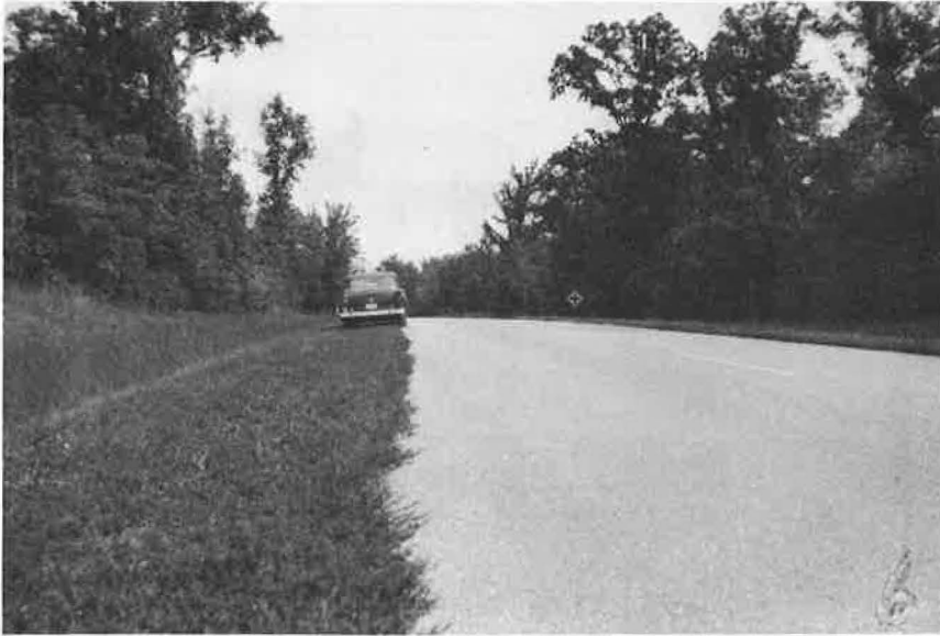
Figure 8. See general comments for Figure 7. A lush growth of turf in stabilized shoulders.
