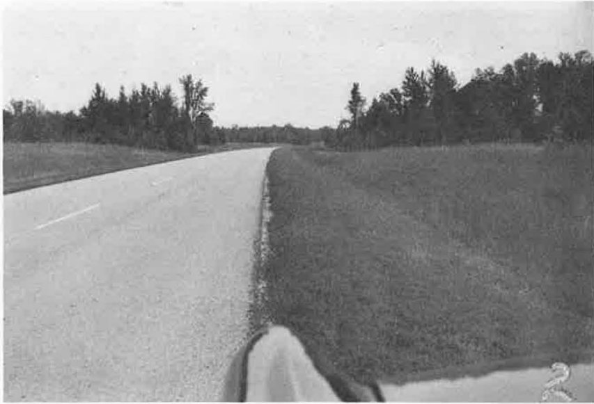
Figure 7. This and Figures 8 and 9 show the varied results on the 6-mile length of the 2A11 portion after three full growing seasons. Photo shows the vestige of the "phantom strip" next to the pavement. The 2A11 portion has a gravel base for the full width of the roadbed.
