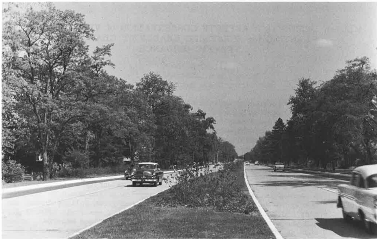
Figure 1. View east along Route 29 Freeway, Trenton, N. J. Relatively narrow median of 16 ft provides space for effective headlight glare screen planting as well as contributing to the attractiveness of the Freeway. The 28-ft separator between main roadway and service or marginal road produces an effective buffer planting area against traffic-noise nuisance. (Courtesy of New Jersey State Highway Dept.)
