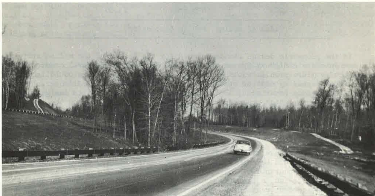
Figure 3. Garden State Parkway. Wide varying median 125 to 130 ft permits adjustment of profiles to fit existing terrain as well as preserving acres of fine wooded areas between roadway that would require years of growing time to replace. (Courtesy of New Jersey State Highway Dept.)
