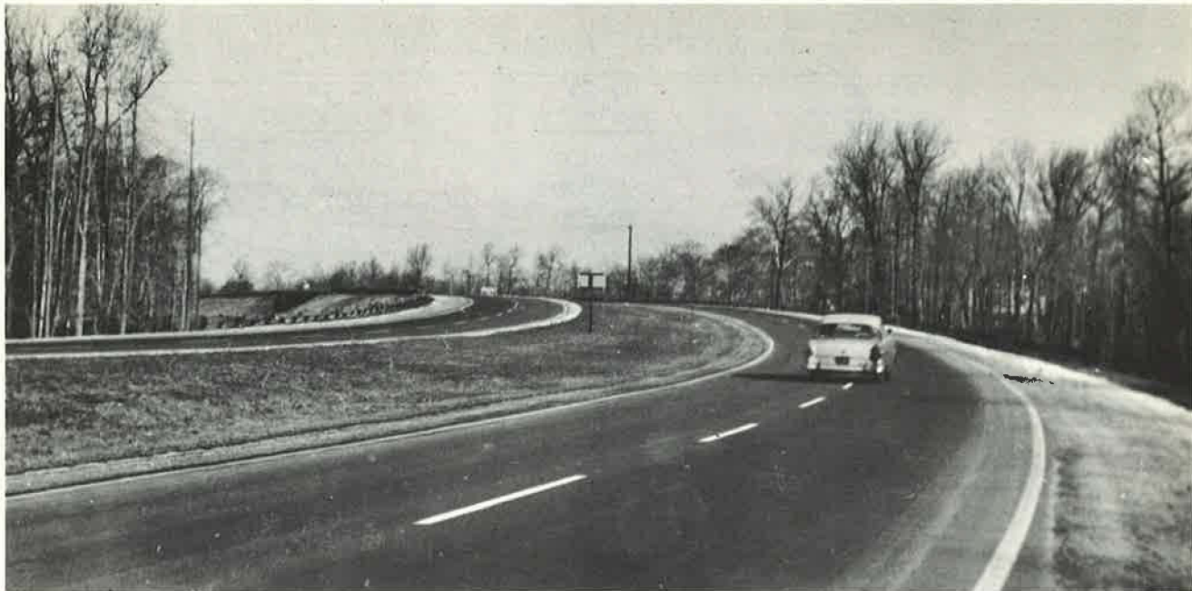
Figure 2. View of Garden State Parkway north of N.J. 4 in Paramus where median is only 29 ft wide. Use of this narrow width at this location made it necessary to remove all existing native growth through this wooded area during construction. (Courtesy of New Jersey State Highway Dept.)
