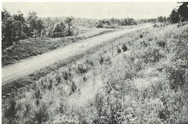
Figure 1. Looking west on Mississippi Highway 30 near Pleasant Ridge Community. The area is hilly, with a highly erosible sandy soil. Pine seedlings were planted in hay mulch in January 1955. Photo was taken in May 1957.
