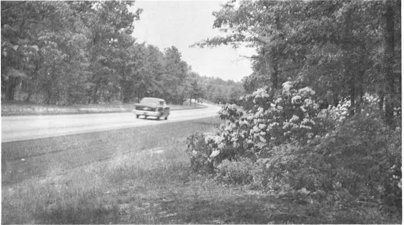
Figure 2. View of a fine stand of native mountain laurel preserved along N.J. Route 70 during construction. Such plant material may be salvaged and moved economically to new locations to help enhance the highway roadside.
