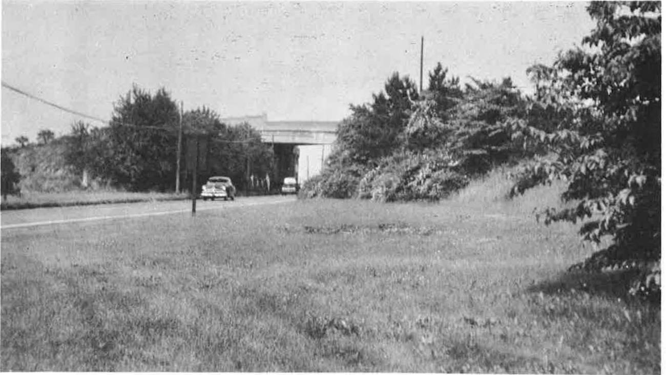
Figure 3. US 130 in the vicinity of Heightstown, New Jersey where a well-designed roadside planting of native vines, shrubs, and trees helps stabilize this high bridge approach fill.
