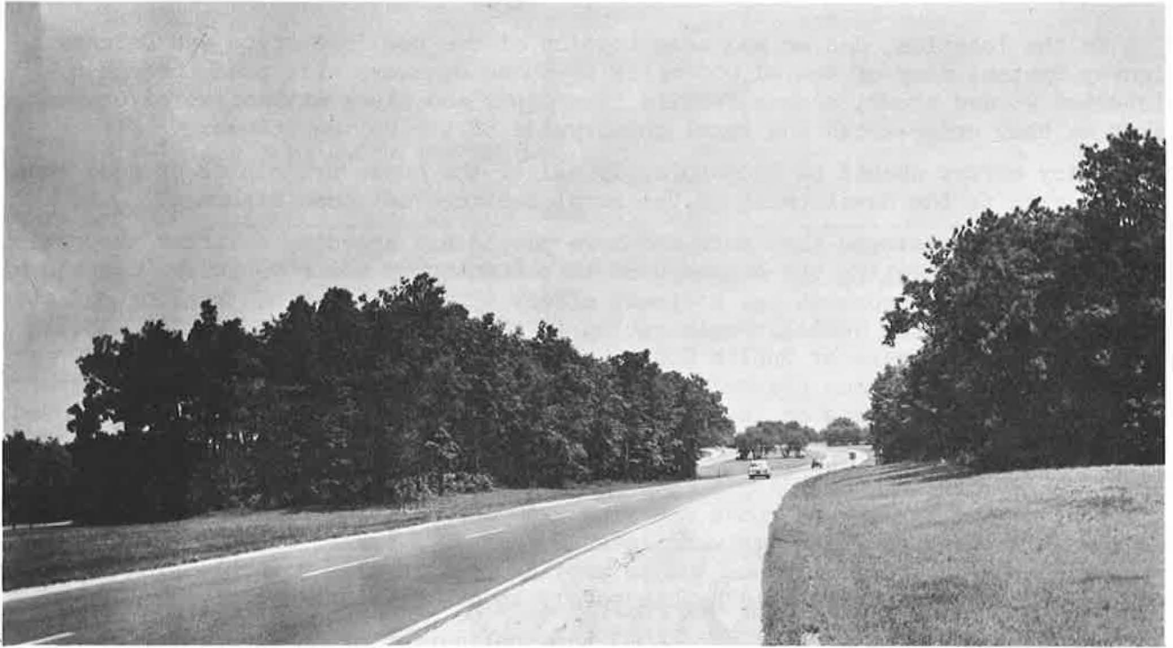
Figure 1. A flowing curvilinear highway alignment usually fits into the existing topography more easily. Conservation of existing tree growth creates a more interesting roadside which helps relieve the monotony of high-speed travel.
