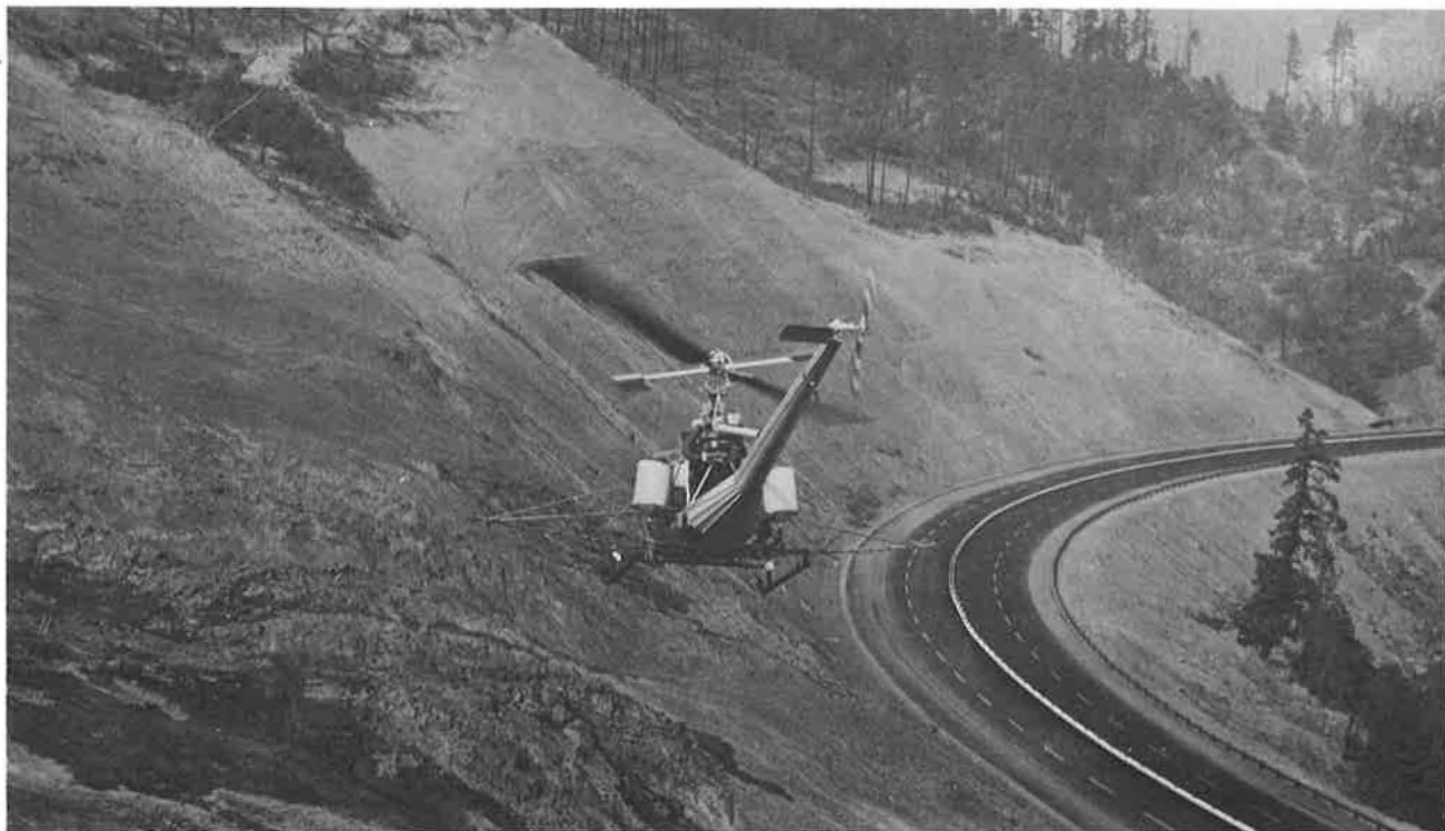
Figure 3. Helicopter flying at about a 50-ft elevation fertilizing the 1:1 cut slopes near Myrtle Creek.
