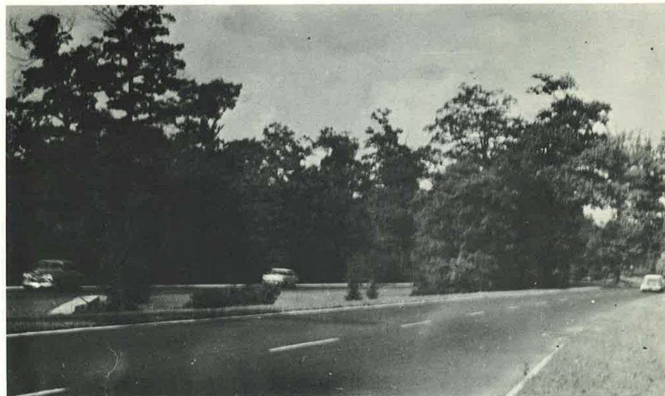
Figure 5. Use of wide median on Palisades Interstate Parkway made it possible to preserve existing native groups of trees and shrubs, which not only eliminate much headlight glare, but also reduce maintenance cost of mowing large grass areas.
