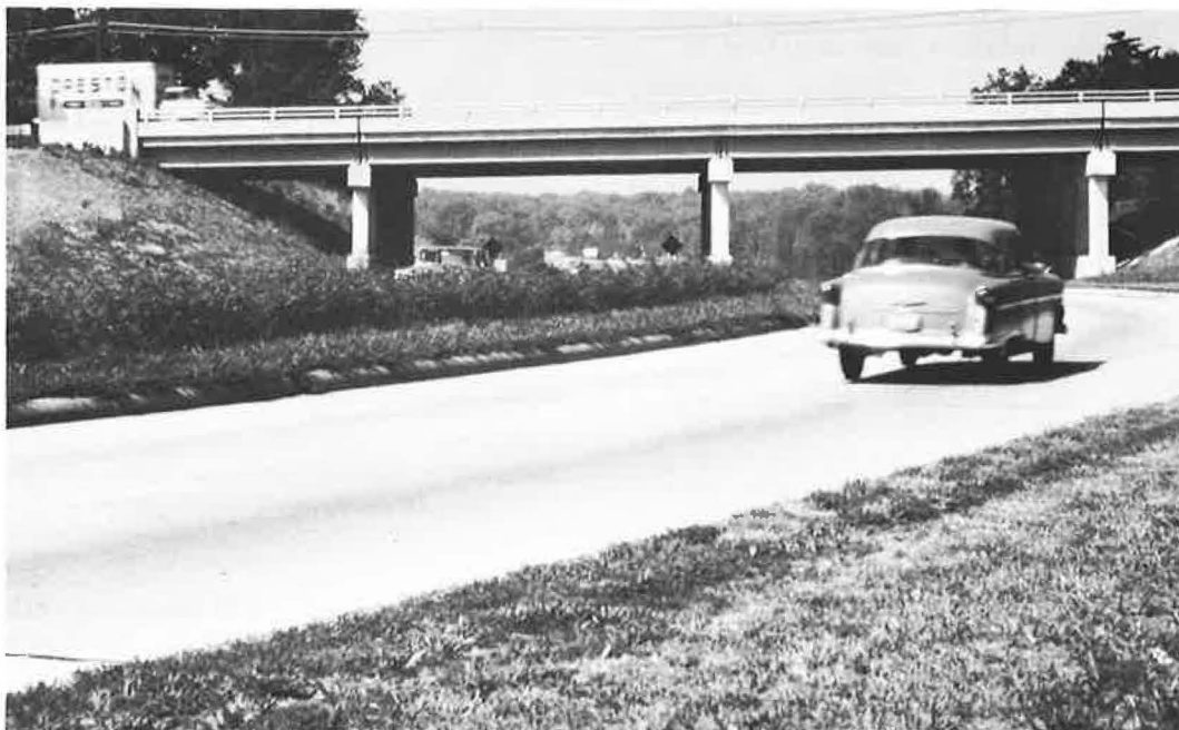
Figure 3. Headlight glare reduction planting, 1960, by Maryland State Roads Commission on Route 193, College Park. Overpass is US 1. Plant material on 15-ft curbed median is Lonicera fragrantissima , nine months after planting.
