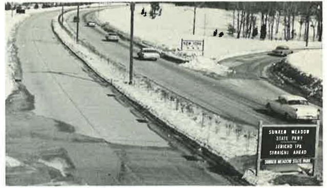
Figure 5. Sunken Meadow Parkway, Long Island, New York. Planting of Crataegus phaenopyrum planted on 5- to 6-ft centers in a 7-ft median.
