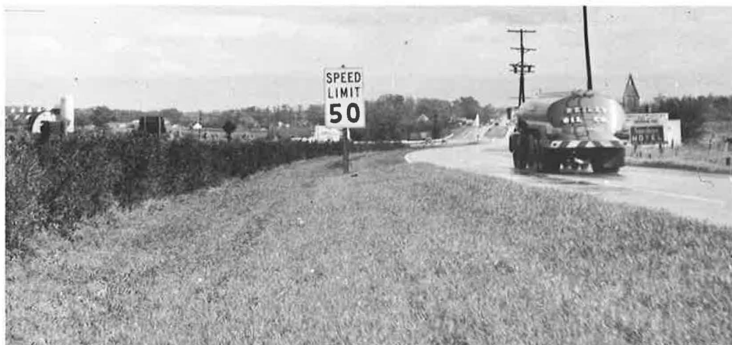
Figure 4. N.J. Route 202, vicinity of Flemington, N.J., where Viburnum prunifolium (Blackhaw) was planted in a double staggered row four foot on centers to screen headlight glare and delineate the changing horizontal alignment. Planting also prevented illegal U-turns of vehicles across the median.
