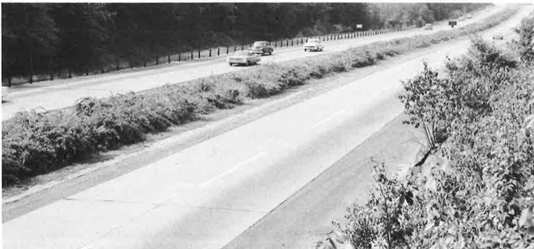
Figure 1. Planting of Rosa multiflora as a headlight-glare screen and crash barrier on Connecticut State Highway.
