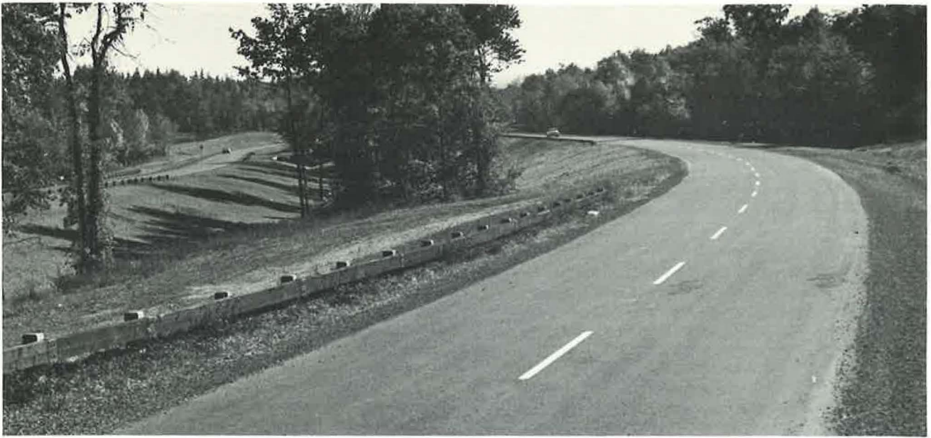
Figure 2. The parkway alignment generally consisted of the curvilinear type which fits the surface of the ground in a series of long flat curves connected by short tangents.
