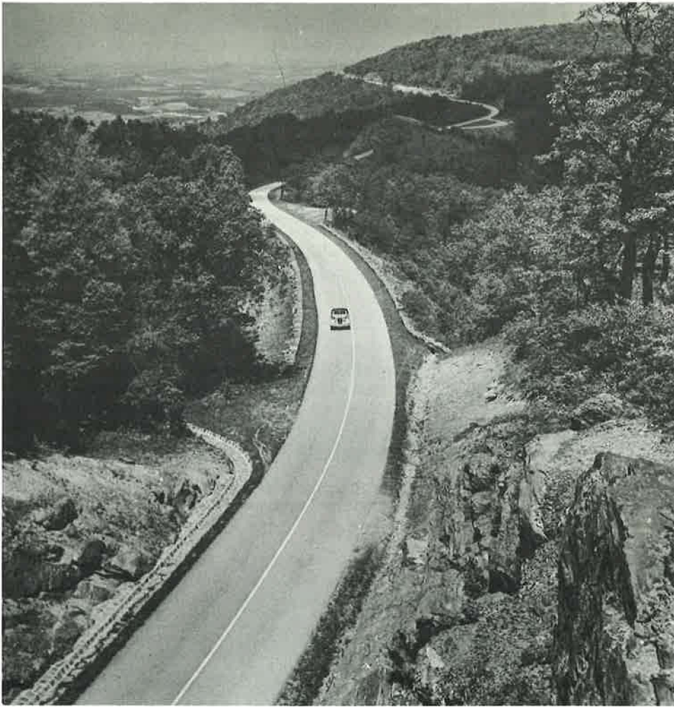
Figure 11. Devils Garden, North Carolina—Parkway road leaves heavy rock cut and skirts edge of escarpment.
