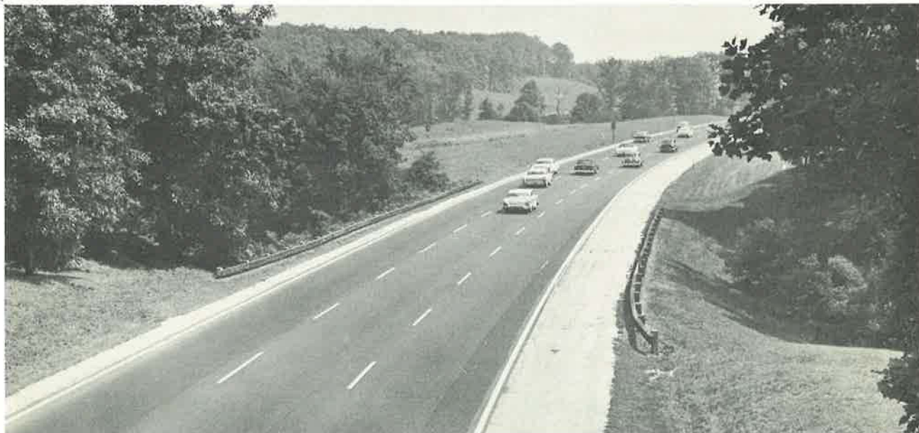
Figure 5. Scenic view of Garden State Parkway looking south over southbound roadway from Nut Swamp Road, Middletown. Northbound roadway in background. Cuts and fills are blended into the existing ground surface by using varying slope grading design standards.
