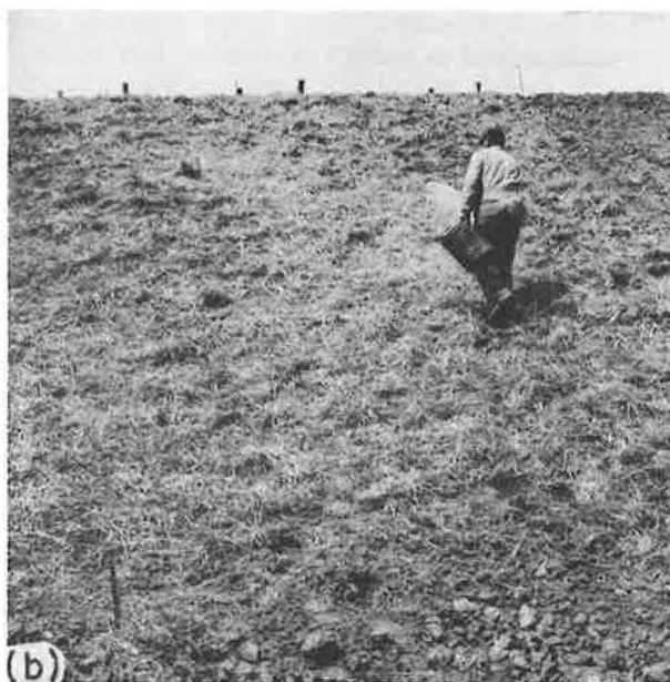
Figure 1. (a) Straw mulch applied by hand at 2 tons per acre. (b) Seed-fertilizer mixture then applied. Seeding of test area (slope depth about 80 ft). Method simulates hydroseeding-straw mulch technique.
