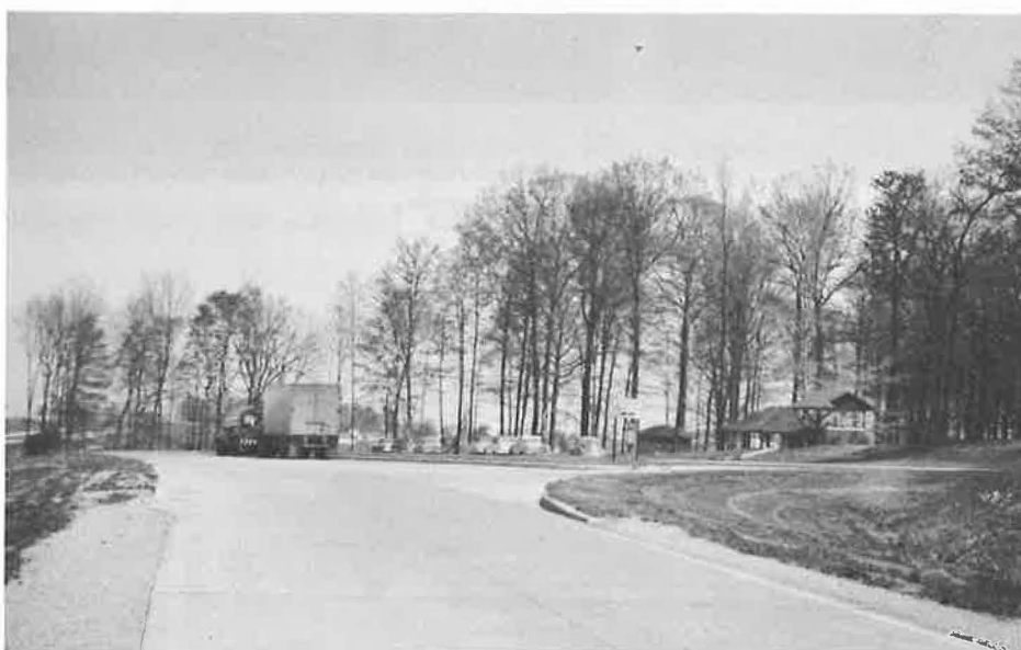
Figure 3. Decelerating lane and truck and car parking areas with planted strip separating the two areas.
