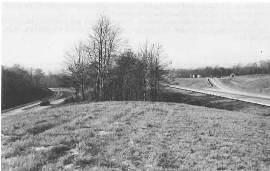
Figure 2. Vegetation in median and the two traffic lanes; decelerating lane and roadside rest on right, accelerating lane and a portion of roadside rest parking area on left.
