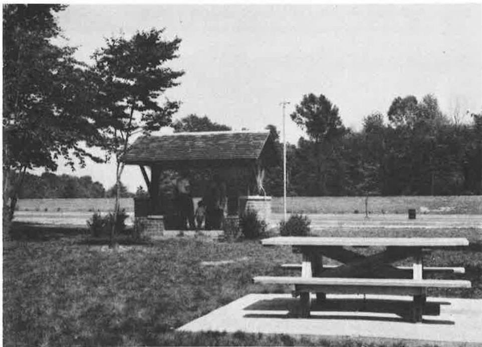
Figure 5. Table on concrete slab, well, and shelter. Note light fixture at right of well shelter.
