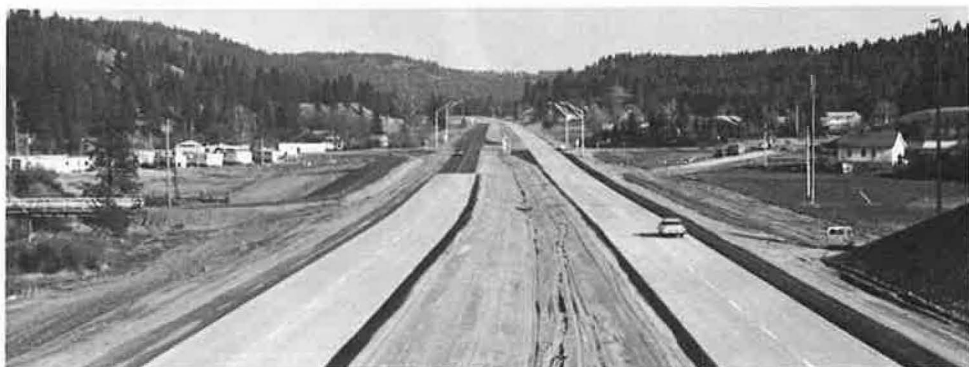
This section of Washington state highway is the scene of the research project on random spacing of joints in portland cement concrete pavements.
