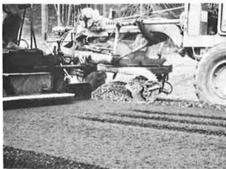
Approximately 4 inches of hot-mix asphalt base was laid in one lift in the APAW-State Highway Commission experiment in 1965. A conventional paver is being used in this photograph, while a motor grader works in the background.
