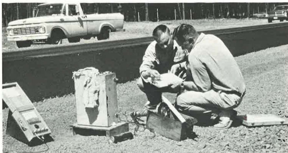
Technicians compare interim test results on one of the thick-lift sections laid in 1965 as a result of the recommendations of the joint research committee.
