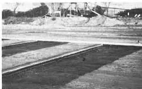
Small bumps in the off-ramp are designed to alert wrong-way drivers without creating a hazard for the driver using the ramp properly.
