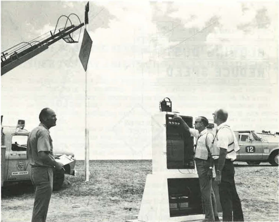
Arizona State Highway Department personnel make final adjustments to the control center of the prototype dust warning signal on Interstate 10. Electronic controls trigger strobe lights on top of pole in background when anemometer (not seen) reaches critical speed.
