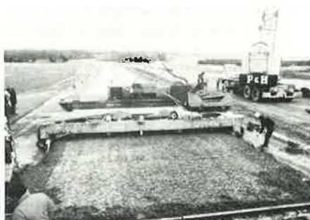
Concrete being spread.
