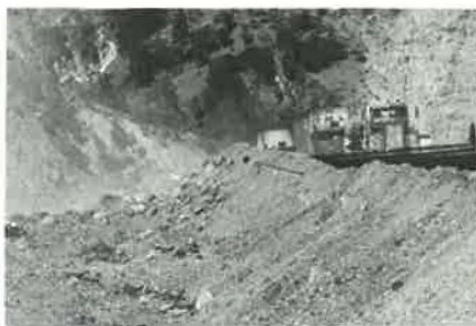
Figure 9. Trench for catching rocks.
