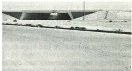
The leveled land seen in the foreground will be the site for one of the large mini-parks slated for construction within the next two years as part of the improvements to I-15 requested by the community. In the background is the new grade separation for D Street, which permits passage under the Interstate route.
