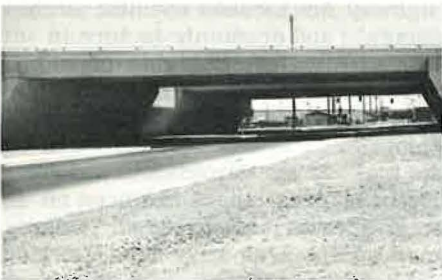
Typical of the new open span structures that provided additional penetrations and kept neighborhoods intact in West Las Vegas is this bridge at F Street.
