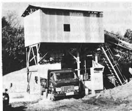
Figure 2. Emulsified asphalt cold-mix plant.
