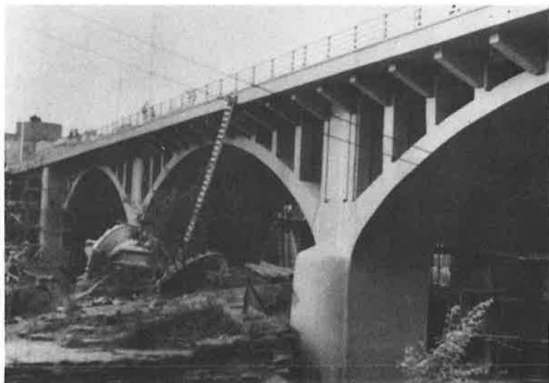
Figure 11. West side of Glens Falls Bridge after being repaired and waterproofed.
