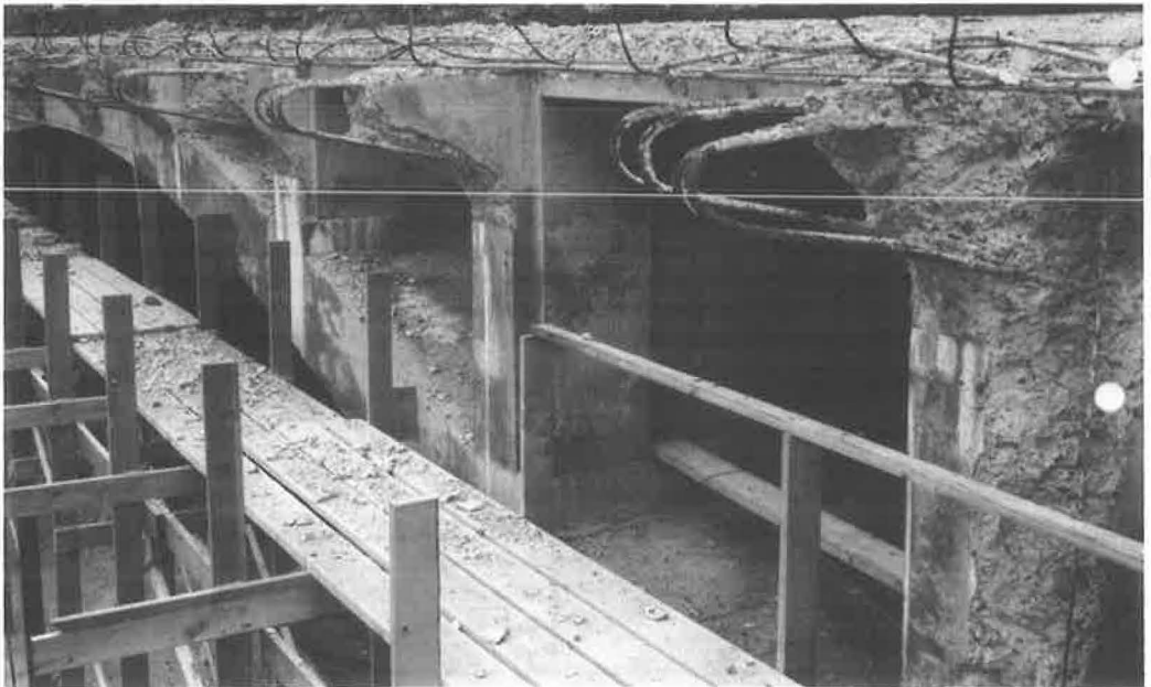
Figure 9. Glens Falls Bridge concrete arches, deteriorated concrete being removed.
