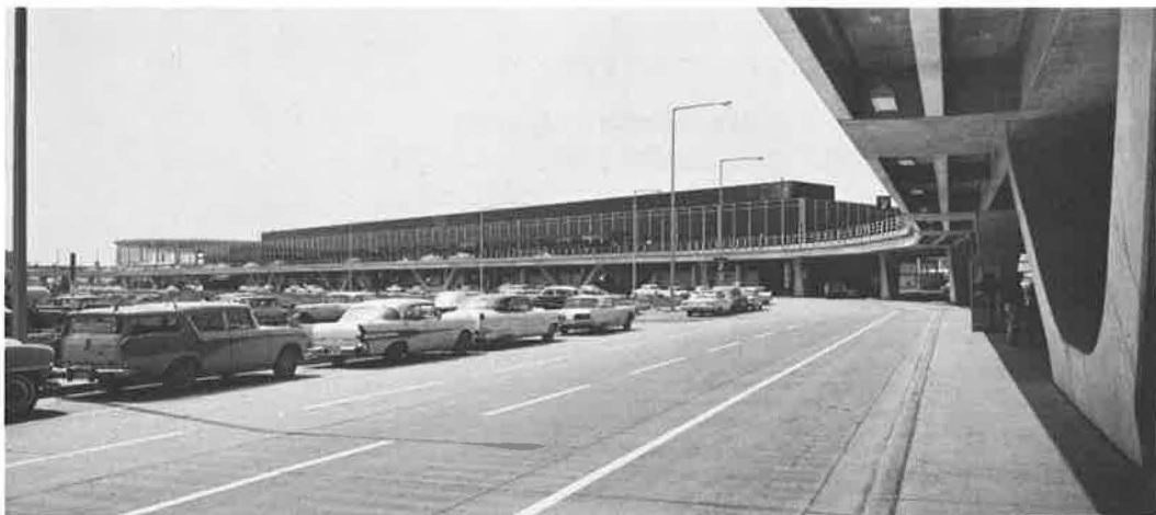
Figure 9. Elevated roadway structure at Chicago's O'Hare Field.
