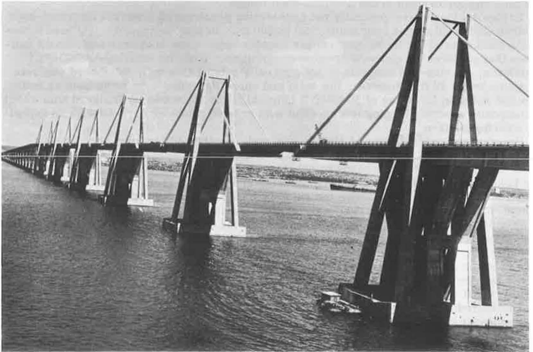
Figure 2. Lake Maracaibo Bridge.
