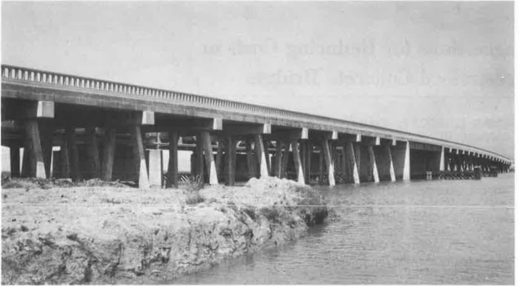
Figure 1. Prestressed flat slab bridge at Eureka, Calif. Spans are 30 ft except for navigation span which is 105 ft composed of post-tensioned I-girders. The piers are of 20-in. square pretensioned square piles.
