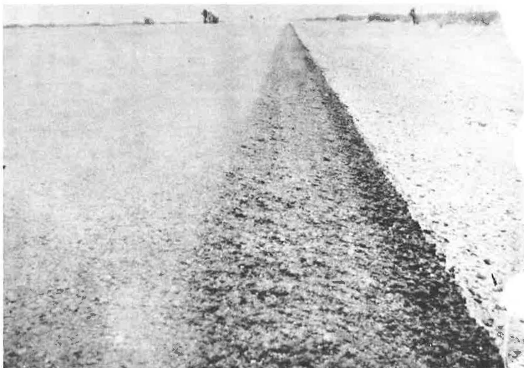
Figure 6. New design shoulder slope, June 21, 1965.
