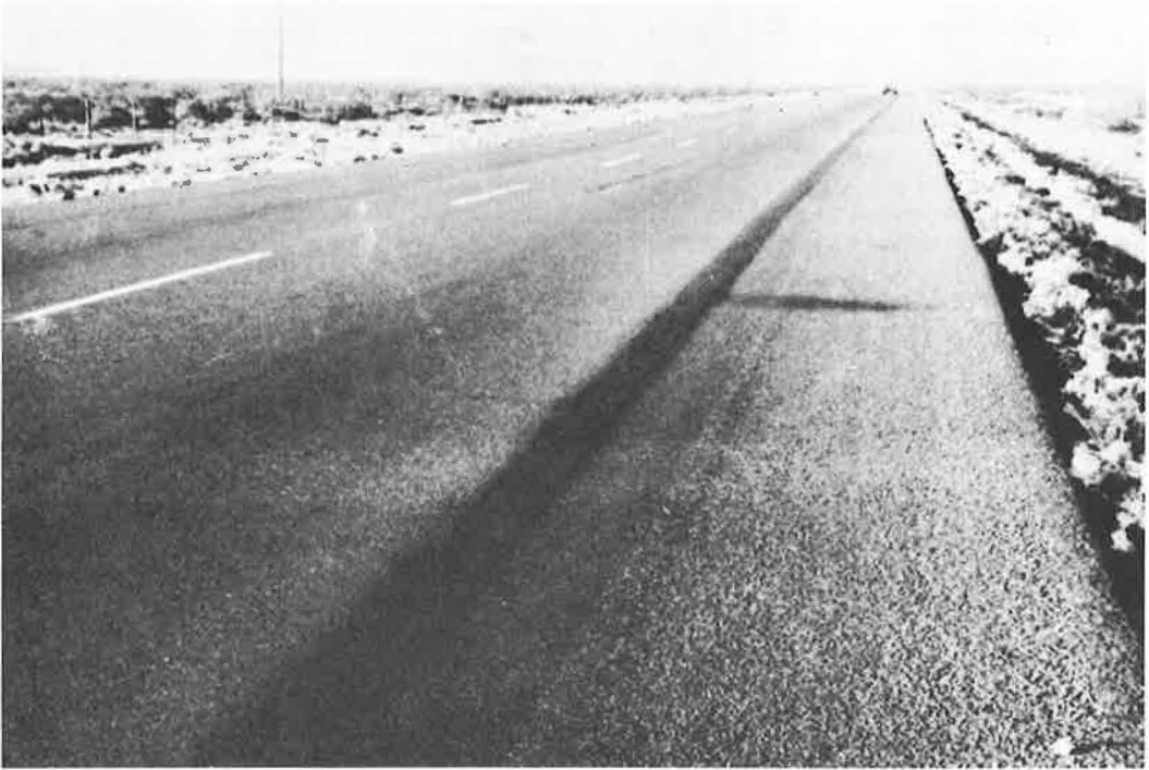
Figure 2. Pavement constructed with crushed limestone, showing little cracking 7 yr after placement.
