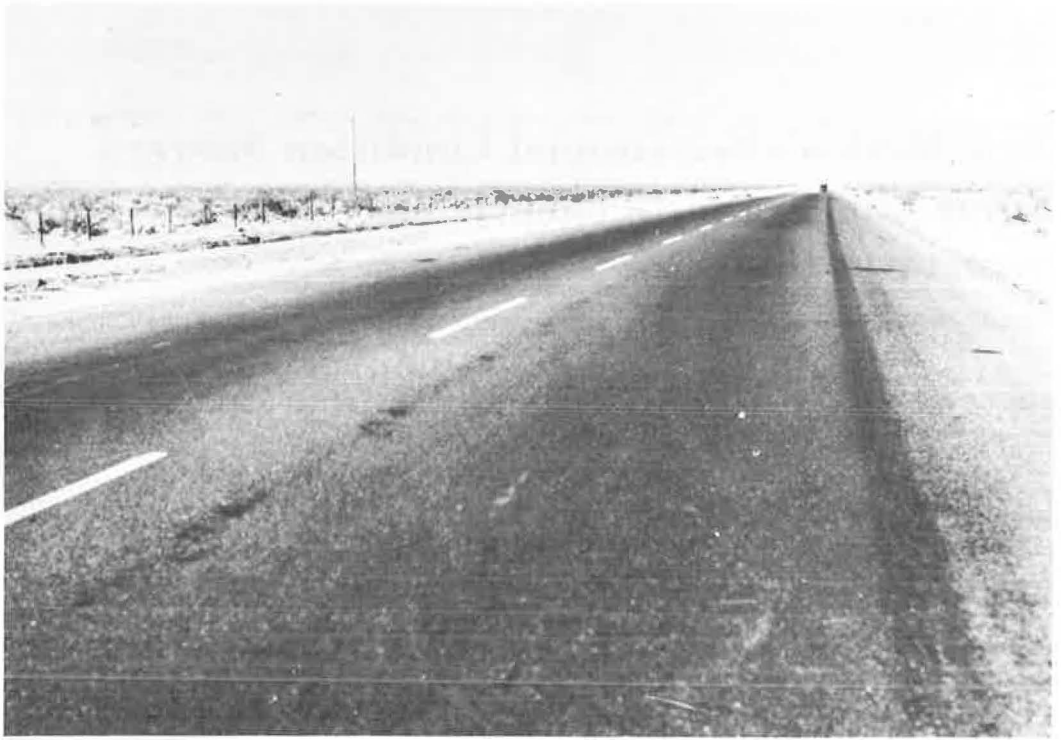
Figure 1. Pavement constructed with crushed limestone, showing little cracking 3 yr after placement.
