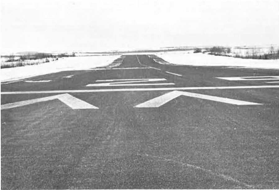
Figure 4. Caribou runway after a 1\frac{1}{2} -in. macadam overlay.
