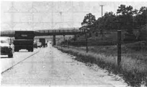
Figure 4. Typical installation of roadside detector.
