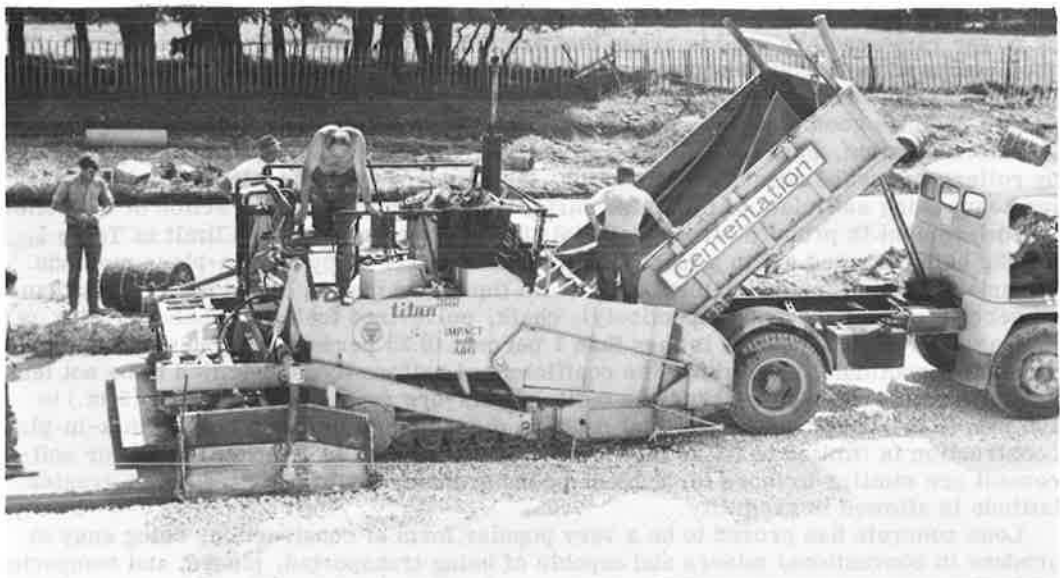
Figure 1. Modified bituminous paver laying cement-stabilized material.
