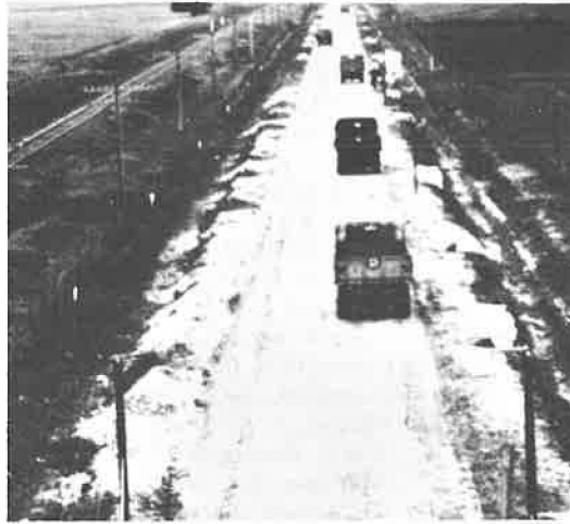
1 One of the earliest full-scale test projects carried out in the United States was the Bates Road Test, which was conducted in Illinois from 1920 until 1923. Fred Burggraf and A.C. Benkelman, who were both to become prominent in HRB activities, participated in the project.
