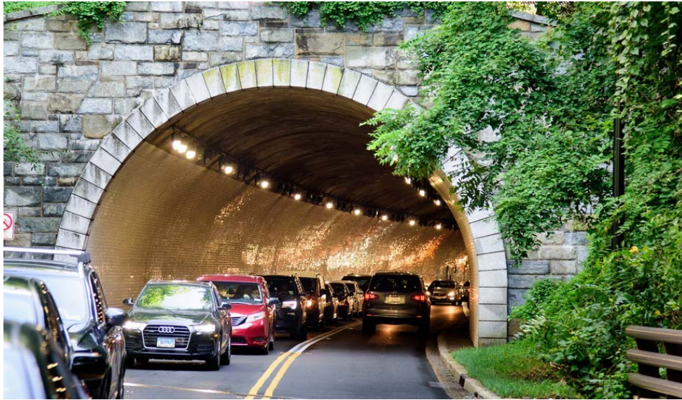
Figure 4-1. Example of a Vehicular Tunnel
