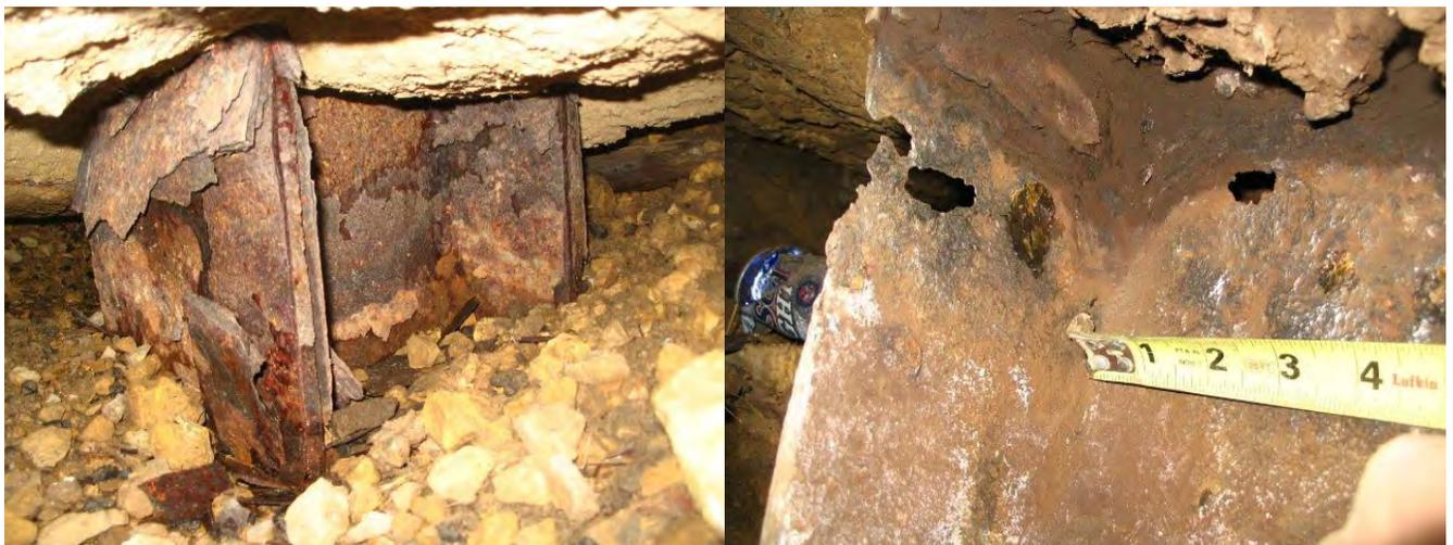
**Figure 54 Iowa DOT Pile Corrosion Example**
