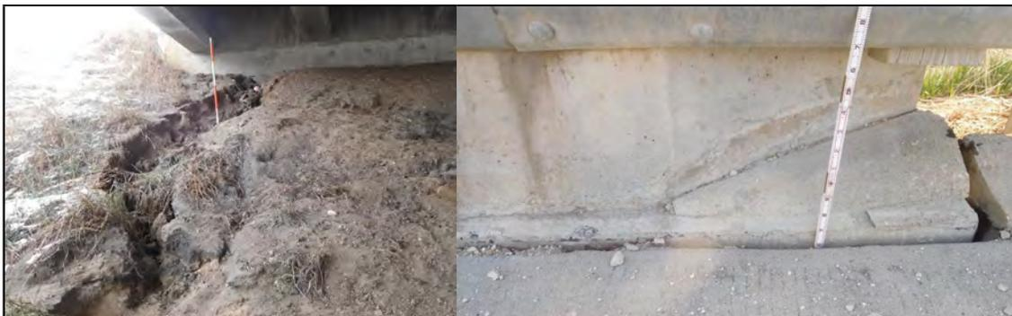
**Figure 47 Iowa DOT Berm Erosion**
