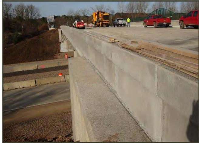
*Figure 7 MnDOT Semi-Integral Abutment with Barrier on top of Approach Panel*
