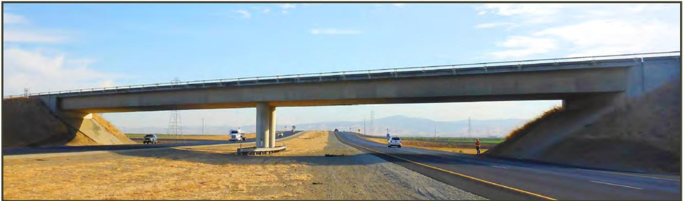
*Figure 2 Caltrans Typical Bridge with Diaphragm Abutments*
