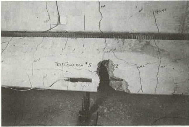
a. East Side of Girder
