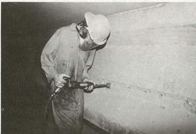
a. Holes Drilled and Surface Being Roughened
