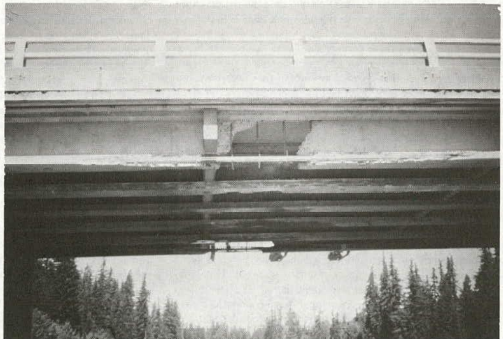
Figure 6. Major concrete damage with no apparent strand damage. (Courtesy of State of Washington DOT)
