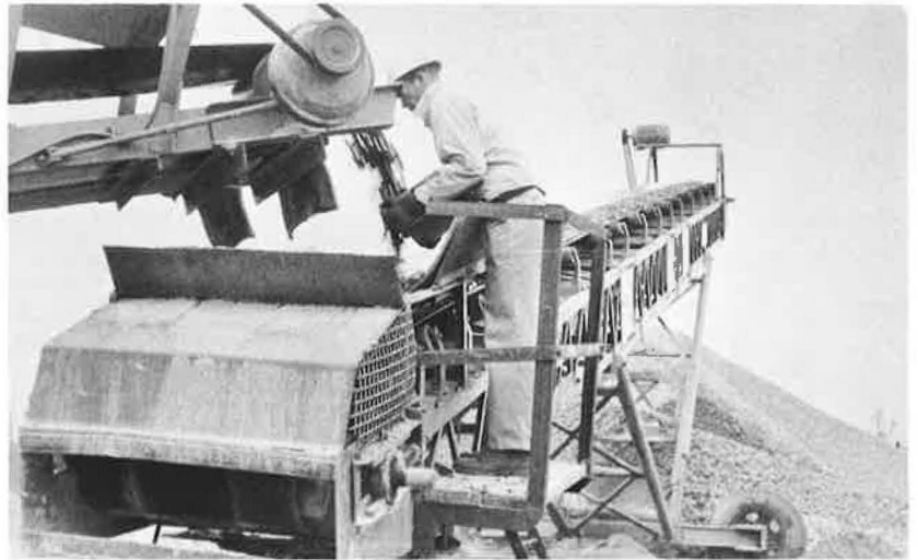
Figure 14. Belt from crusher to stockpile in Series No. 3. Test portions were obtained by passing a metal container through the stream of aggregate as in lower picture. This aggregate was subsequently hauled to an asphalt plant located about \frac{1}{4} mile from the stockpile area.
