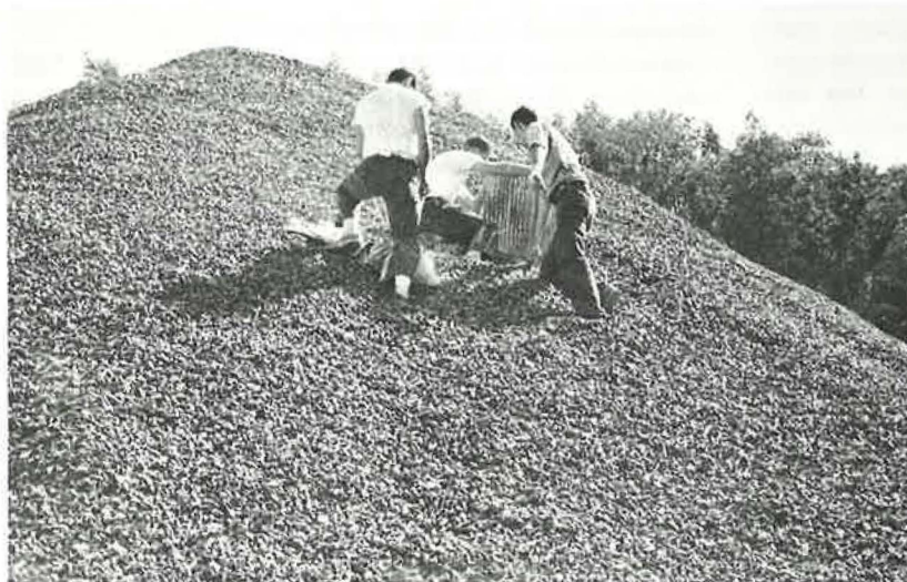
Figure 12. Some typical problems facing an inspector charged with the duty of taking a meaningful sample from a mountainous stockpile.
