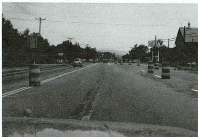
Figure 3.39. Use of barrels at a Case C restricted work zone.
