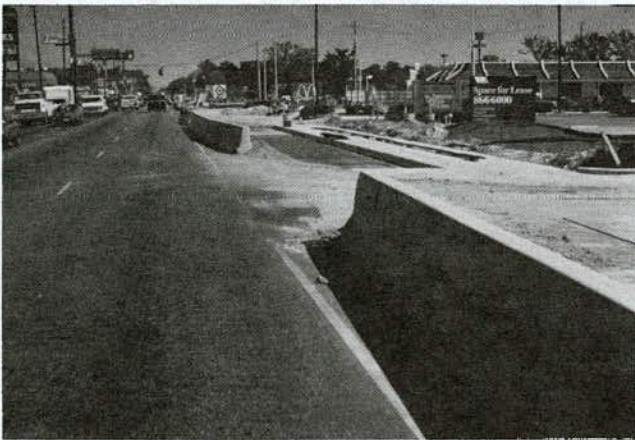
Figure 2.8. Barrier openings for access at a Case C restricted work zone. (Note: Treatments shown in Figures 2.8 and 2.9 are not necessarily recommended.)
