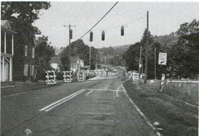
Figure 3.7. Barricades placed at the end of the barrier.
