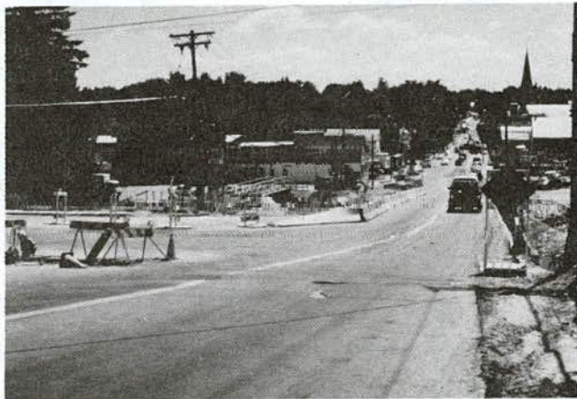
Figure 3.3. Sloped-end treatment at a Case B restricted work zone.
