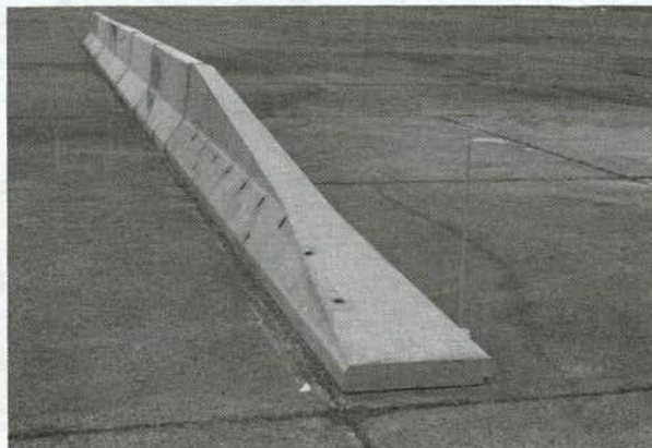
FIGURE IV-4. PHOTOS OF CONVENTIONAL SLOPED-END TREATMENT USED IN TEST PROGRAM
