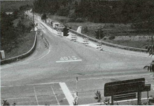
Figure 2.6. Case B restricted work zone at a T-intersection.
