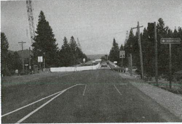
Figure 3.1. Barrier flared at a steeper rate than standard. (Note: Treatments shown in Figures 3.1 to 3.7 are not necessarily recommended.)
