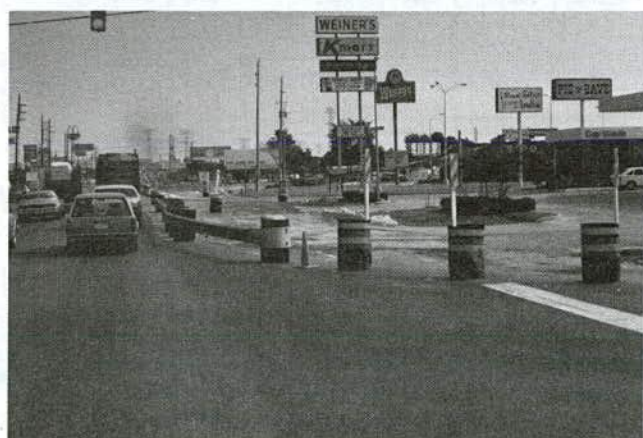
Figure 3.38. W-beam-on-barrels "wrapped around" at access drives and roadways.
