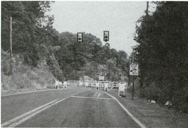
Figure 3.6. Traffic detour to a temporary roadway.
