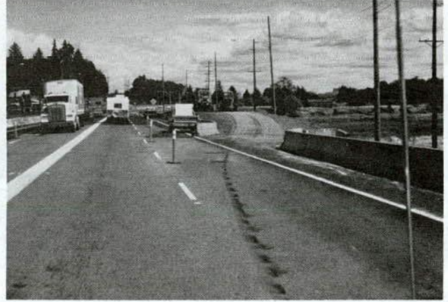
Figure 2.9. Temporary barrier opening for contractor access at a Case C restricted work zone.
