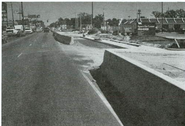
Figure 3.37. Temporary concrete barrier placed along roadway at a Case C restricted work zone. (Note: Treatments shown in Figures 3.37 and 3.39 are not necessarily recommended.)
