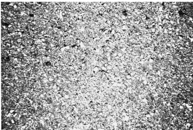
Figure 10. Popouts and raveling in 2-year-old pavement.
