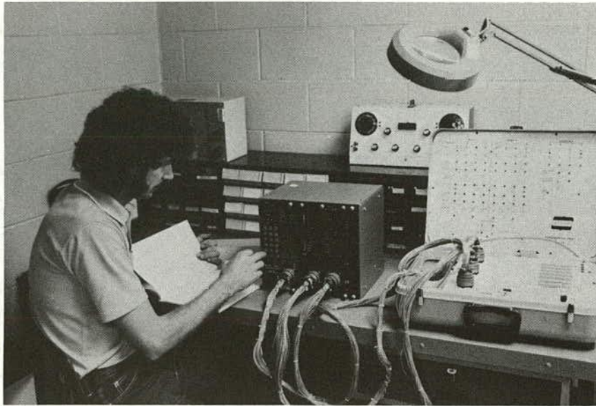
FIGURE 3 Technician using NEMA test board with a controller in Macon.
